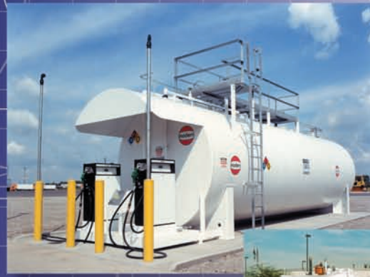
Dispensing Diesel Fuel With 20,000 Gallon Fireguard Tank
