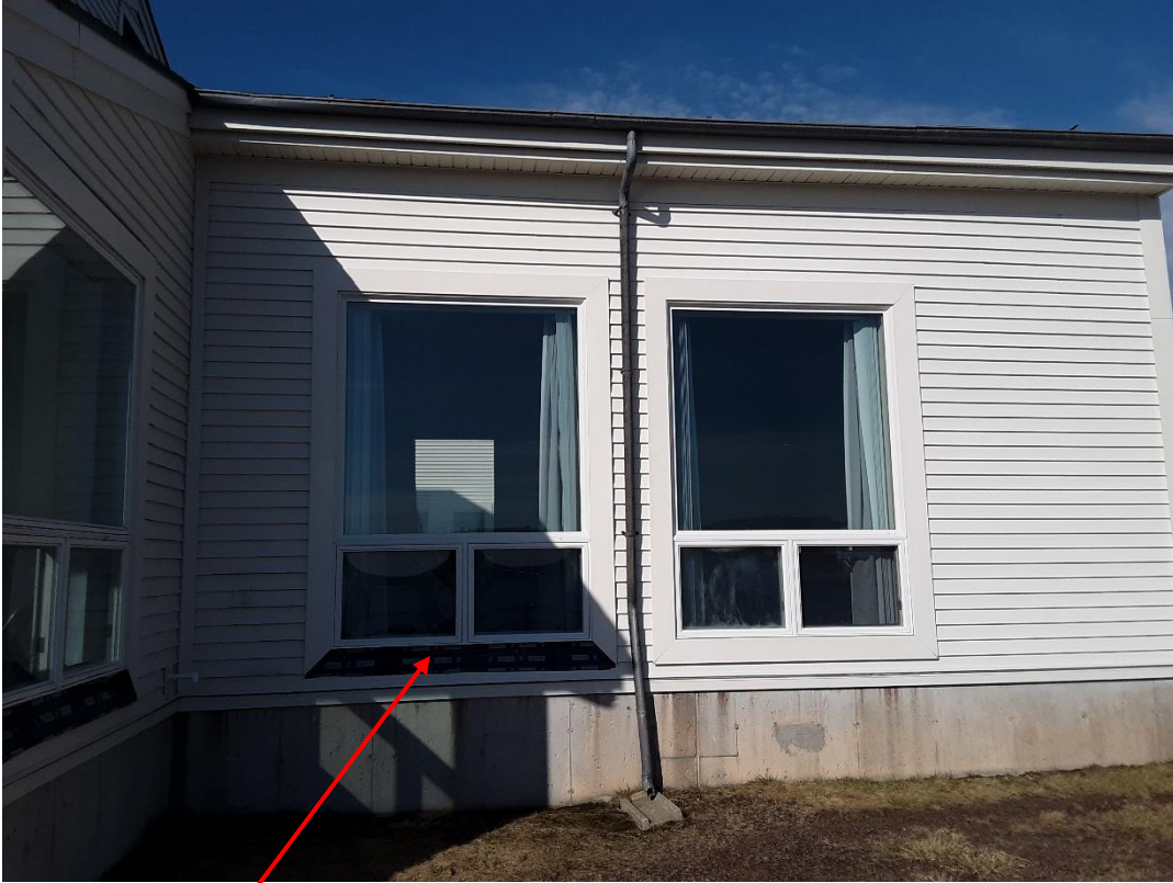
This is the north end conference room windows which are 8.6 feet high and are 6 feet wide. Missing trim.
