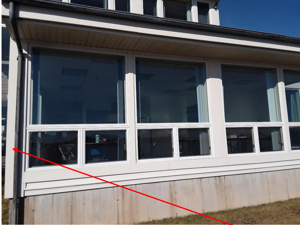
These windows are 7.6 feet high and 6 feet wide. There are seven of these windows. Please note where arrow is a corner trim piece which will need replacement also and has a different length.
