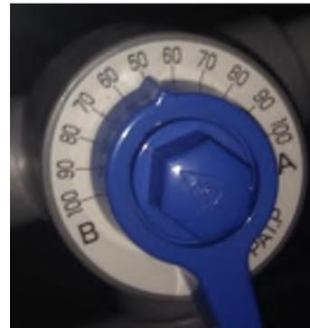
**9. Check/Set Effluent Airlift Valve (white).**
