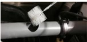
**15. Refill the chlorinator (if applicable).** Place refill chlorination tablets in the chlorinator tube and adjust the dissolve rate by rotating the bottom cap of the chlorinator.
