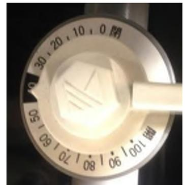
At start-up, and for standard operation, the Effluent Airlift Valve (white) should be set to 40%. 18
