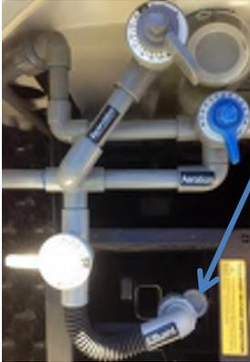
**14. Clean Recirculation Air-lift Pump (Recommended frequency: 1x every 6 months)**
