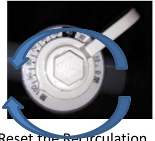
**H.** Reset the Recirculation Control Valve (grey valve) and the Effluent Control Valve (white valve) to their original positions. Make sure that the aeration is working properly.
