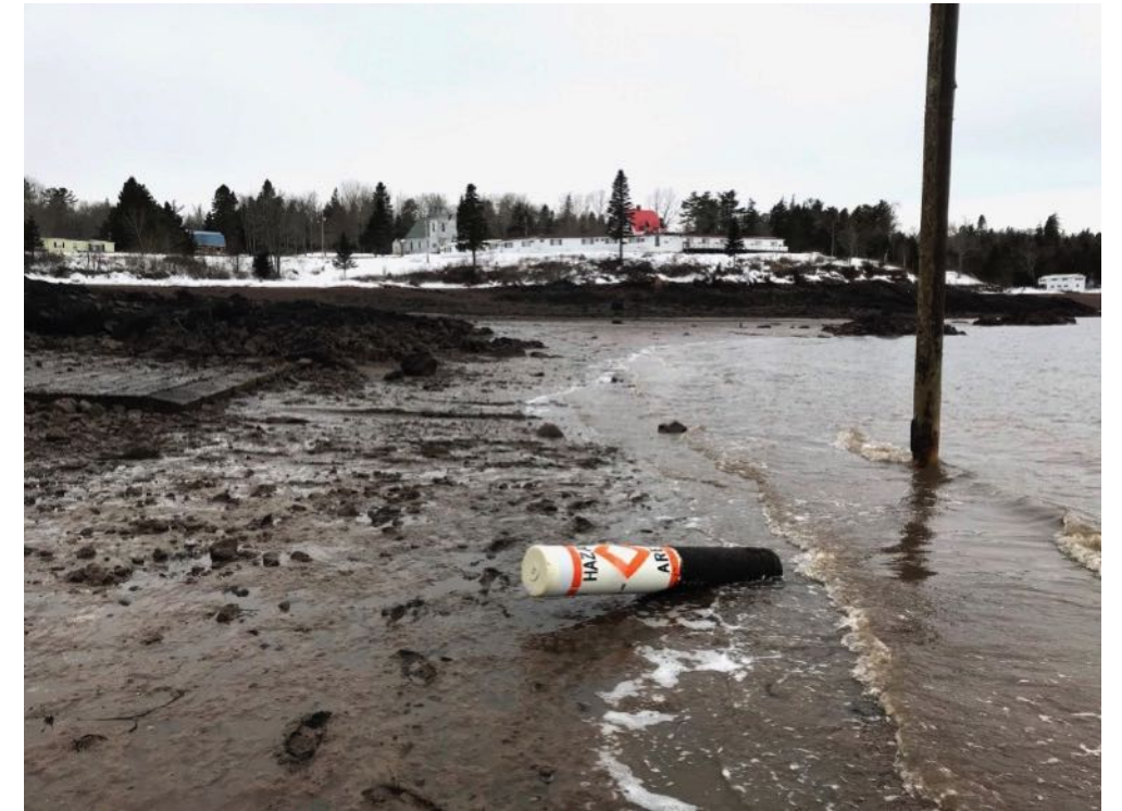
Pile #9 and end of ramp
