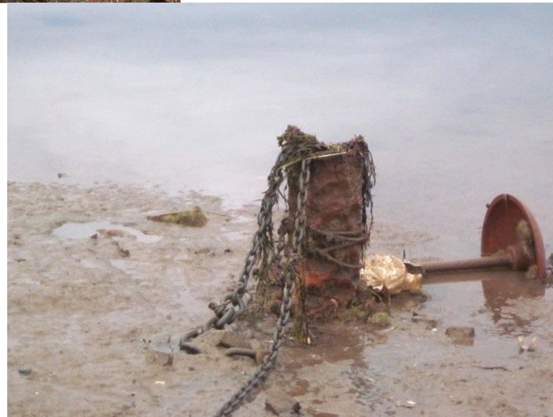
Pile #10 remaining stub, photo taken at low drain tide
