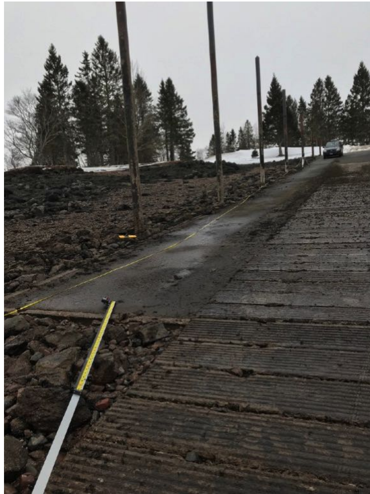
End of paved float laydown area. Pile #7 is first pile on the left
