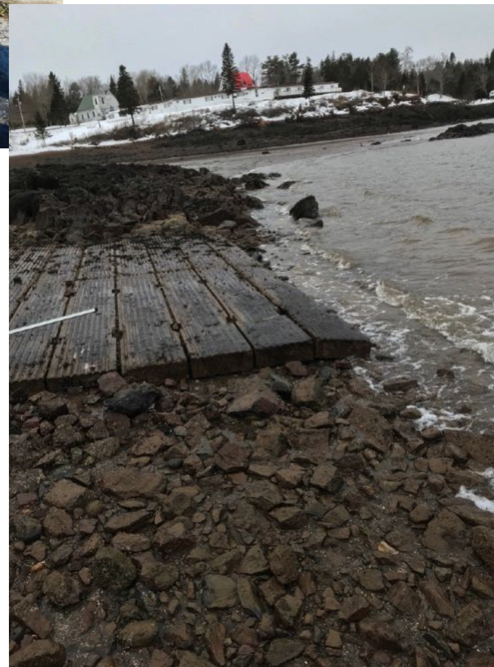
End of ramp planks
