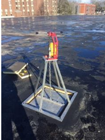
Test area #2 before pulling on assembly
