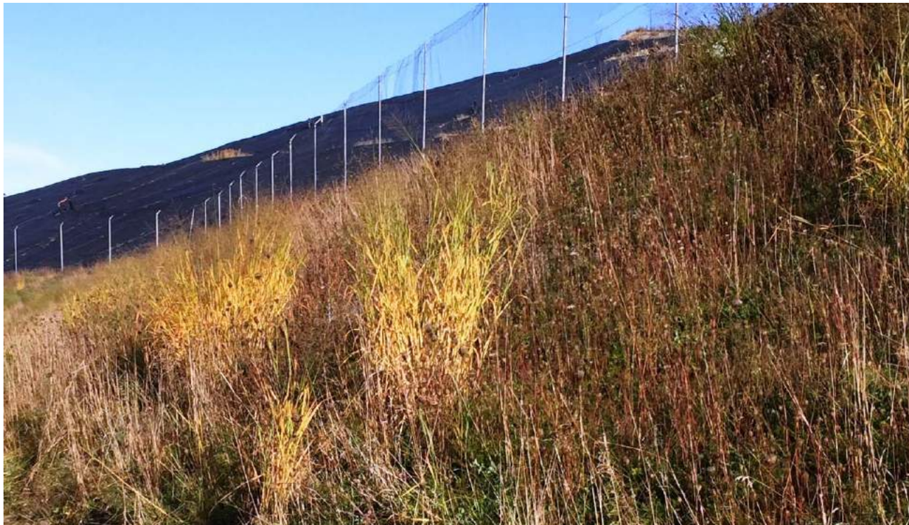
23. south corner looking northwest to southerly slope of Cells 4/5 & lower vegetative slope of Cells 5/6
