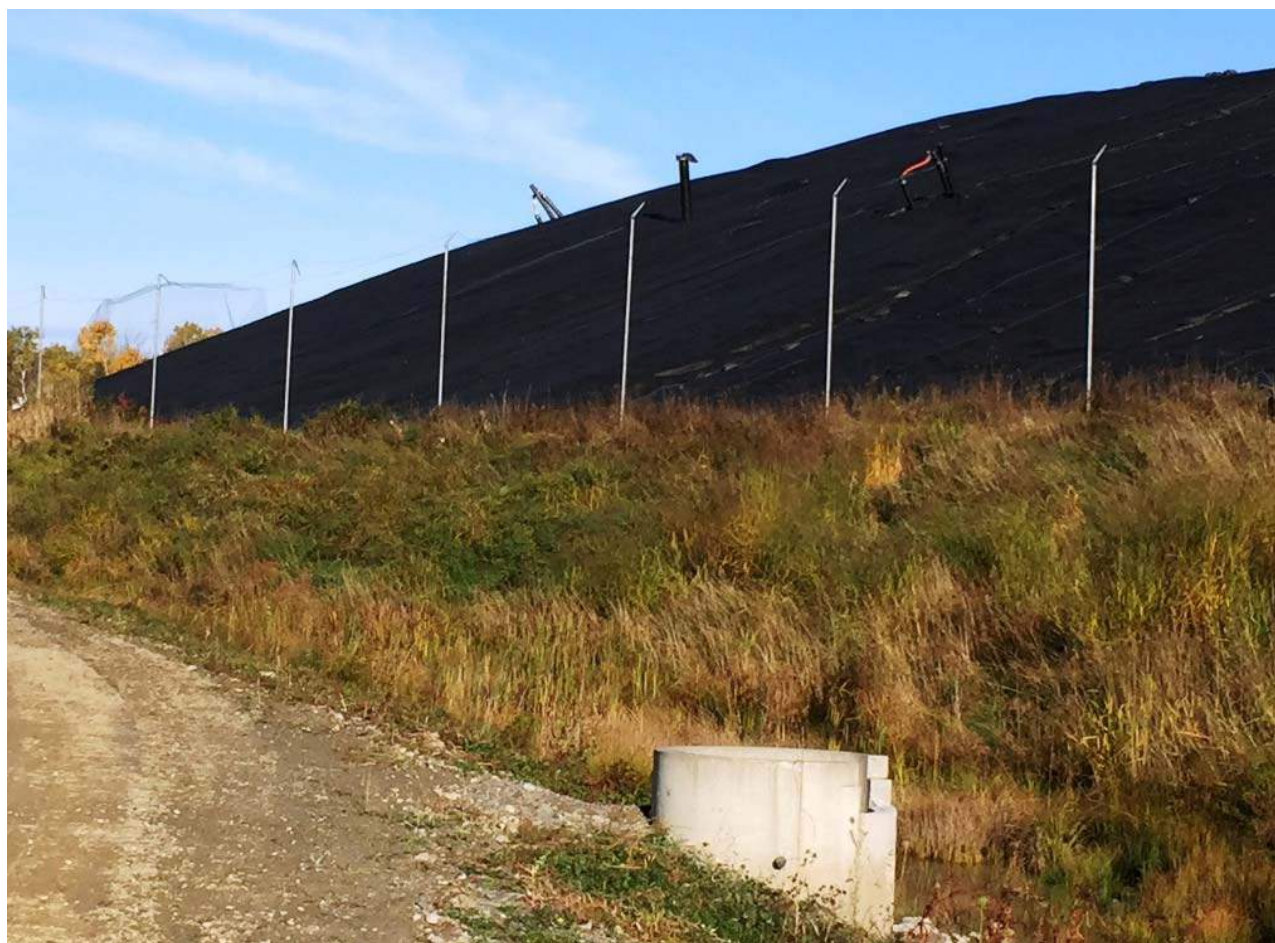
24. southerly slope of Cells 4/5 & lower vegetative slope of Cells 5/6
