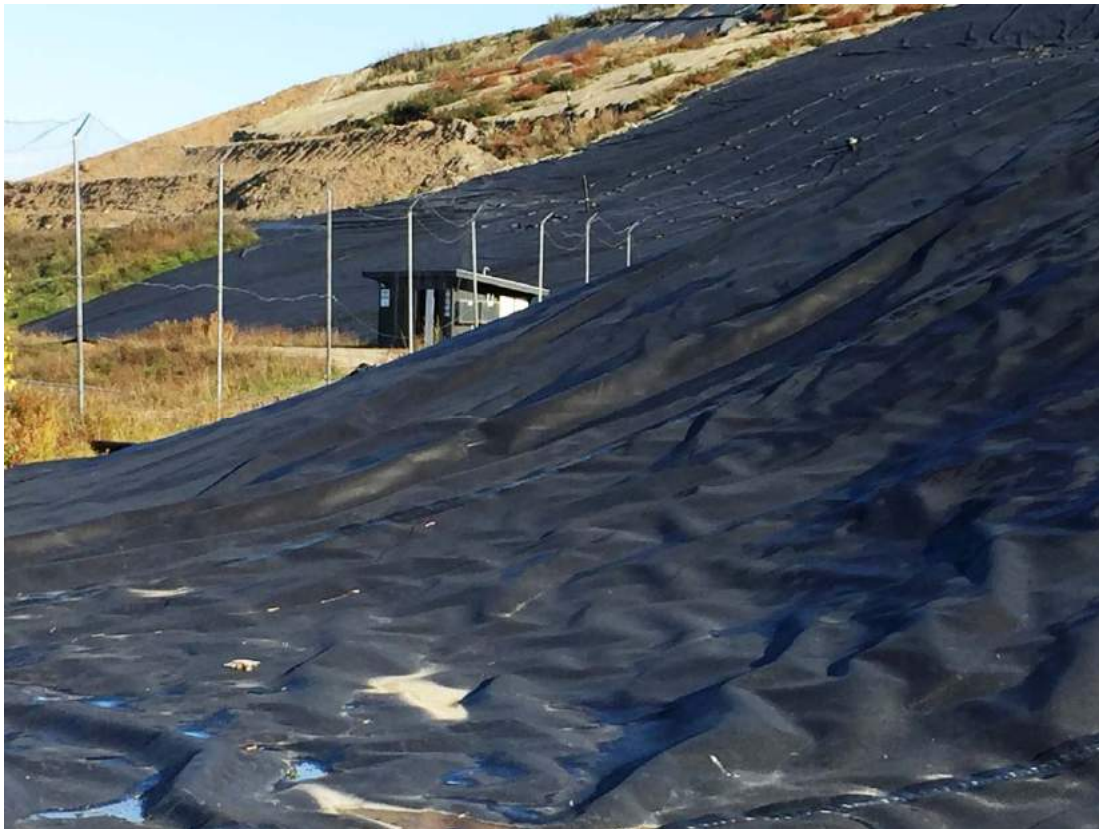
29. southwestern corner looking northeasterly to Cells 1&2 (with excavation area) and lower Cell 4
