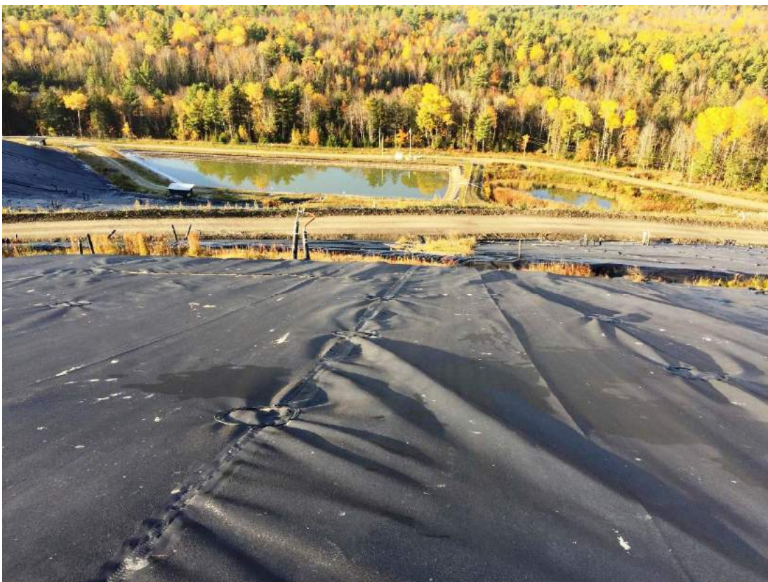
9. landfill top looking down westerly slope of Cell 1 & 2 towards western detention ponds
