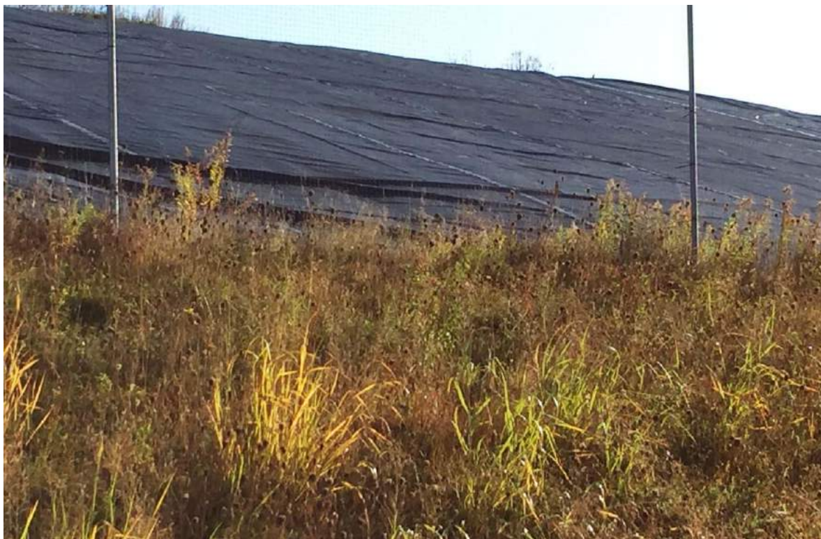
27. looking southeasterly up the southwesterly slope of Cells 5/6
