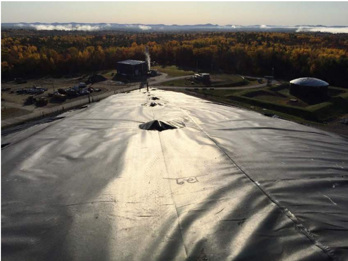
14. looking southeasterly along southeastern ridge line of Cell 9
