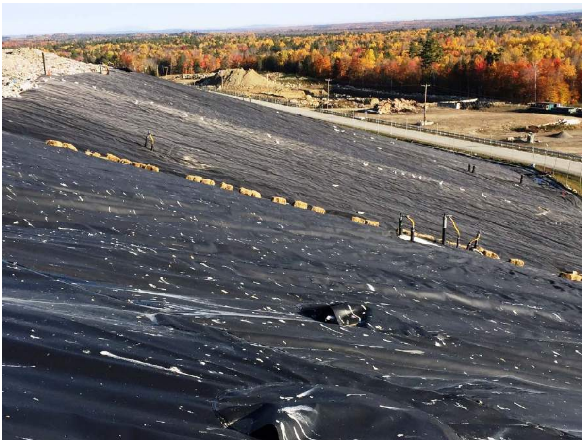
16. on southeasterly ridge line looking northerly along lower eastern slope of Cell 11/9
