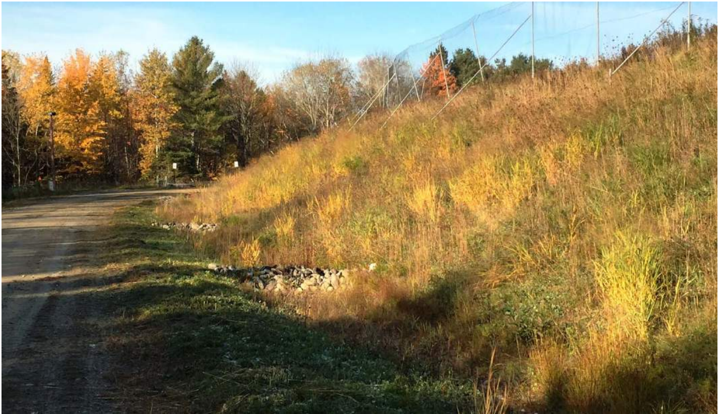
21. southern vegetative slope of Cell 8 & perimeter drainage ditch
