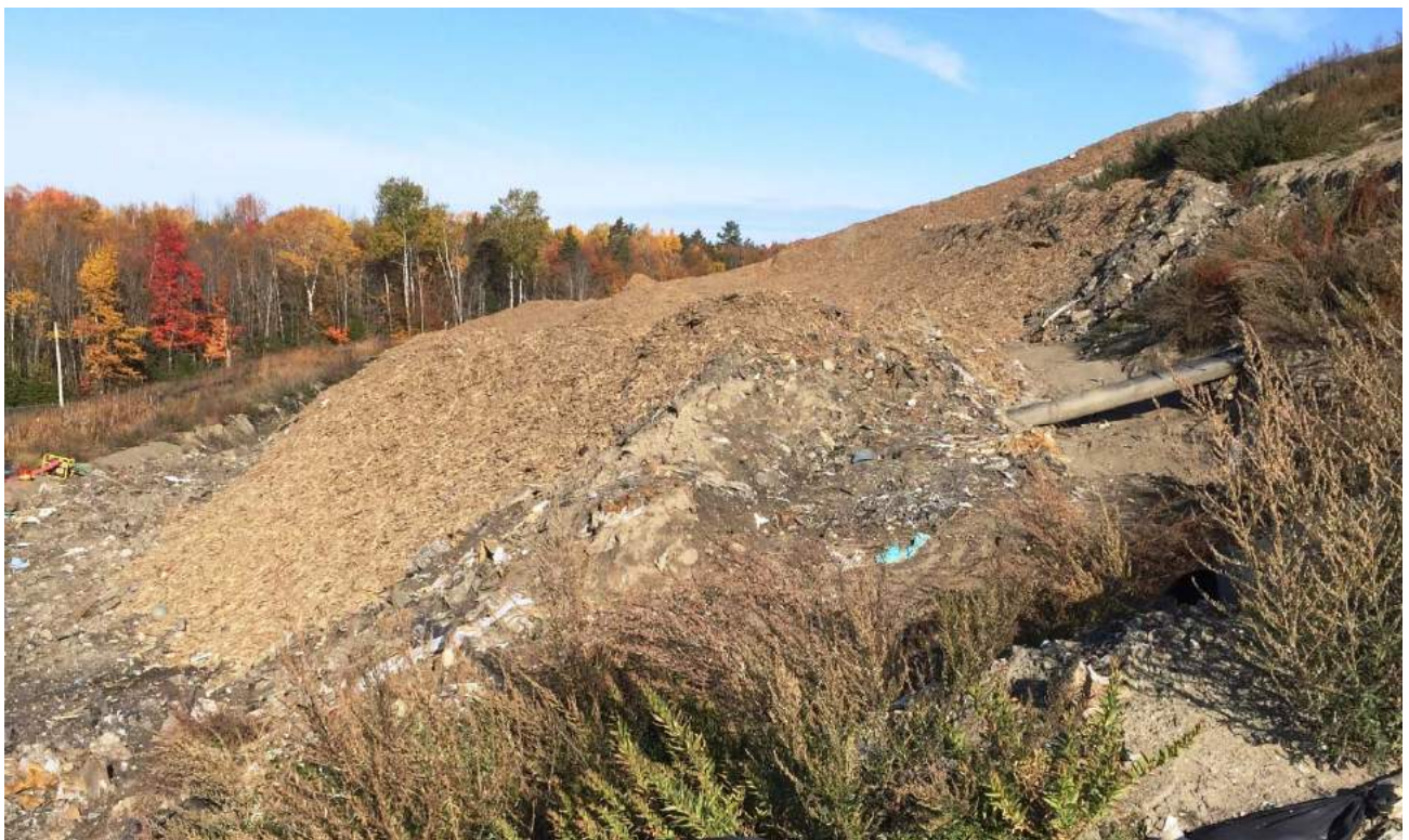
32. excavation area looking northwesterly on the southwesterly slope of Cells 1 & 2
