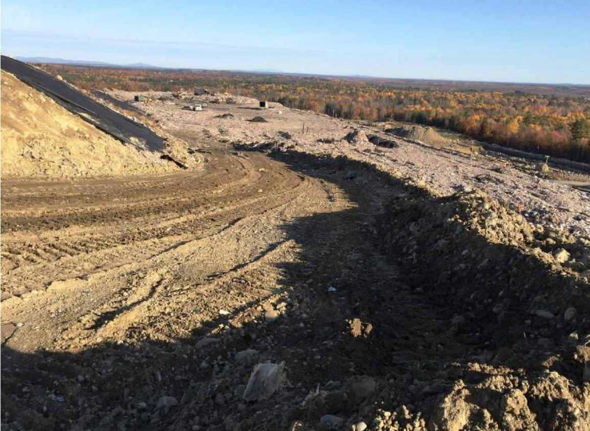
12. top access road to Cell 9 looking northerly along eastern slope of Cell 9 towards Cell 11 operations
