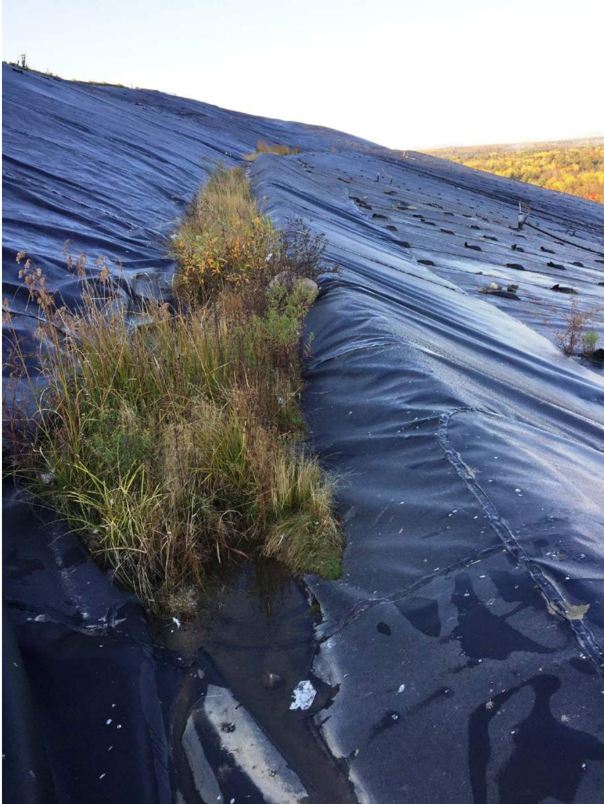
4. northern slope looking southwesterly along transition slope between Cell 3 & Cell 1 & 2
