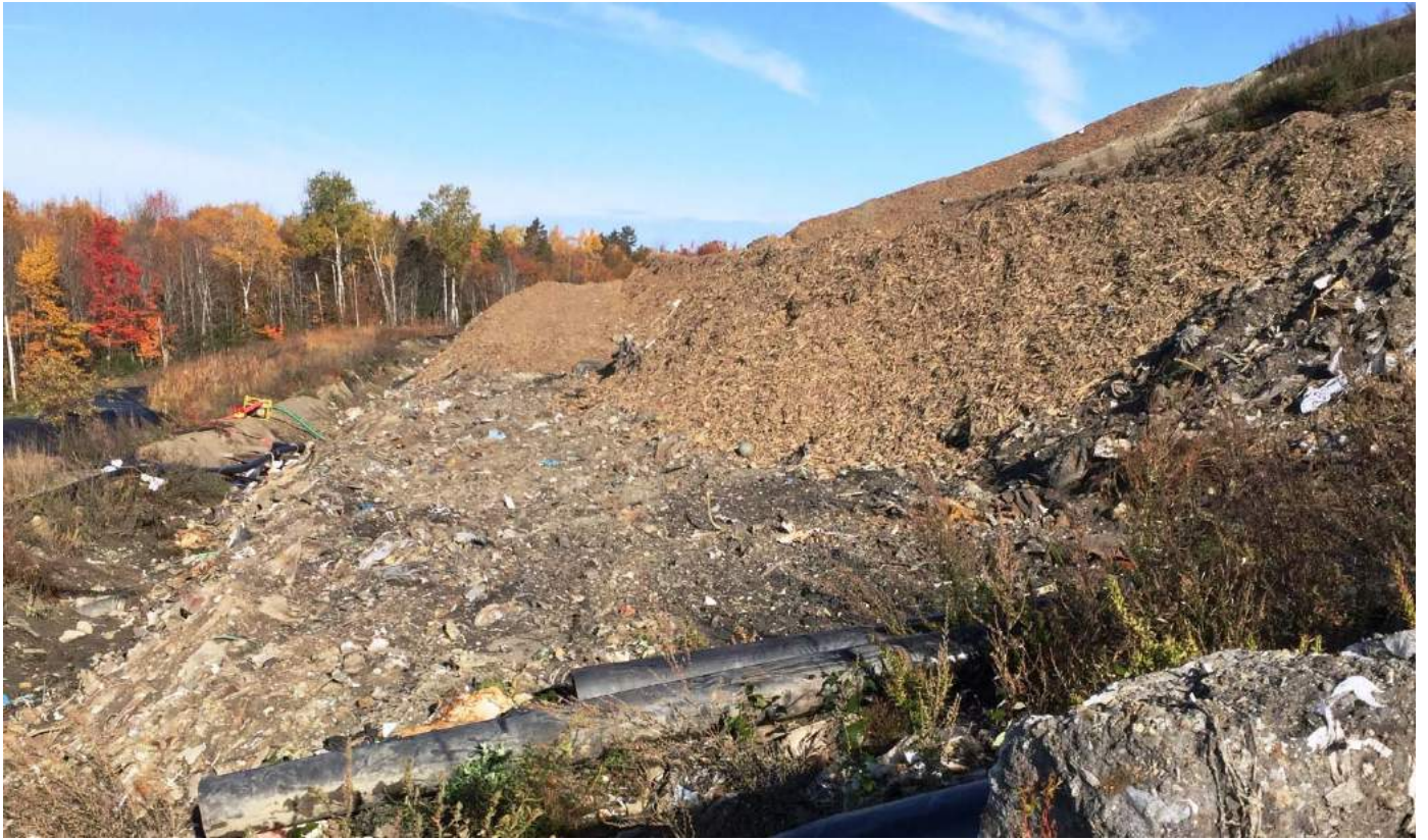
31. excavation area looking northwesterly on the southwesterly slope of Cells 1 & 2
