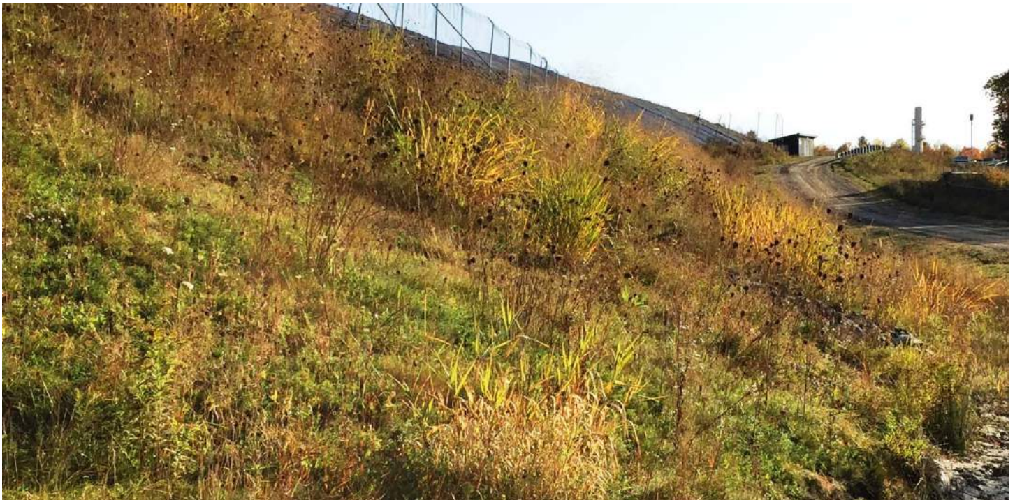
22. south corner looking easterly to southerly vegetative slope of Cells 5/6
