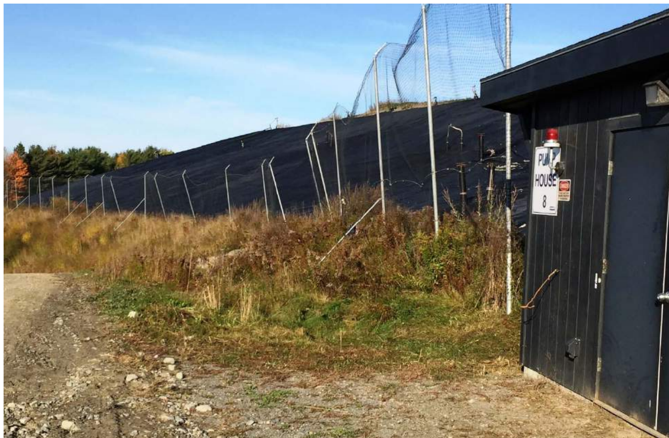
19. at Pump House 8 looking easterly along the lower southern slope of Cells 5/6/8
