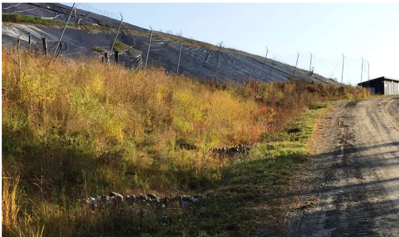
20. west of Pump House 8 looking easterly along Cell 8 south slope of & perimeter drainage ditch
