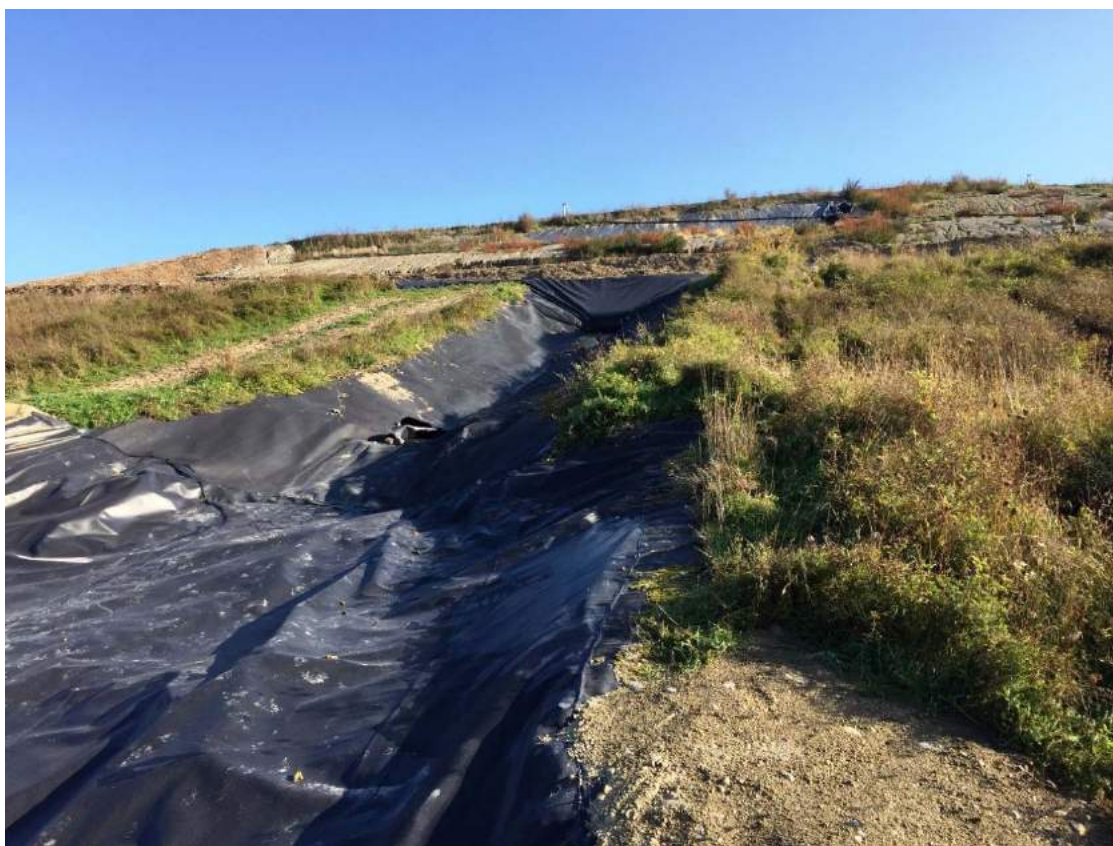
30. at western detention ponds looking easterly up the western slope of Cells 1/2 (towards excavation area)
