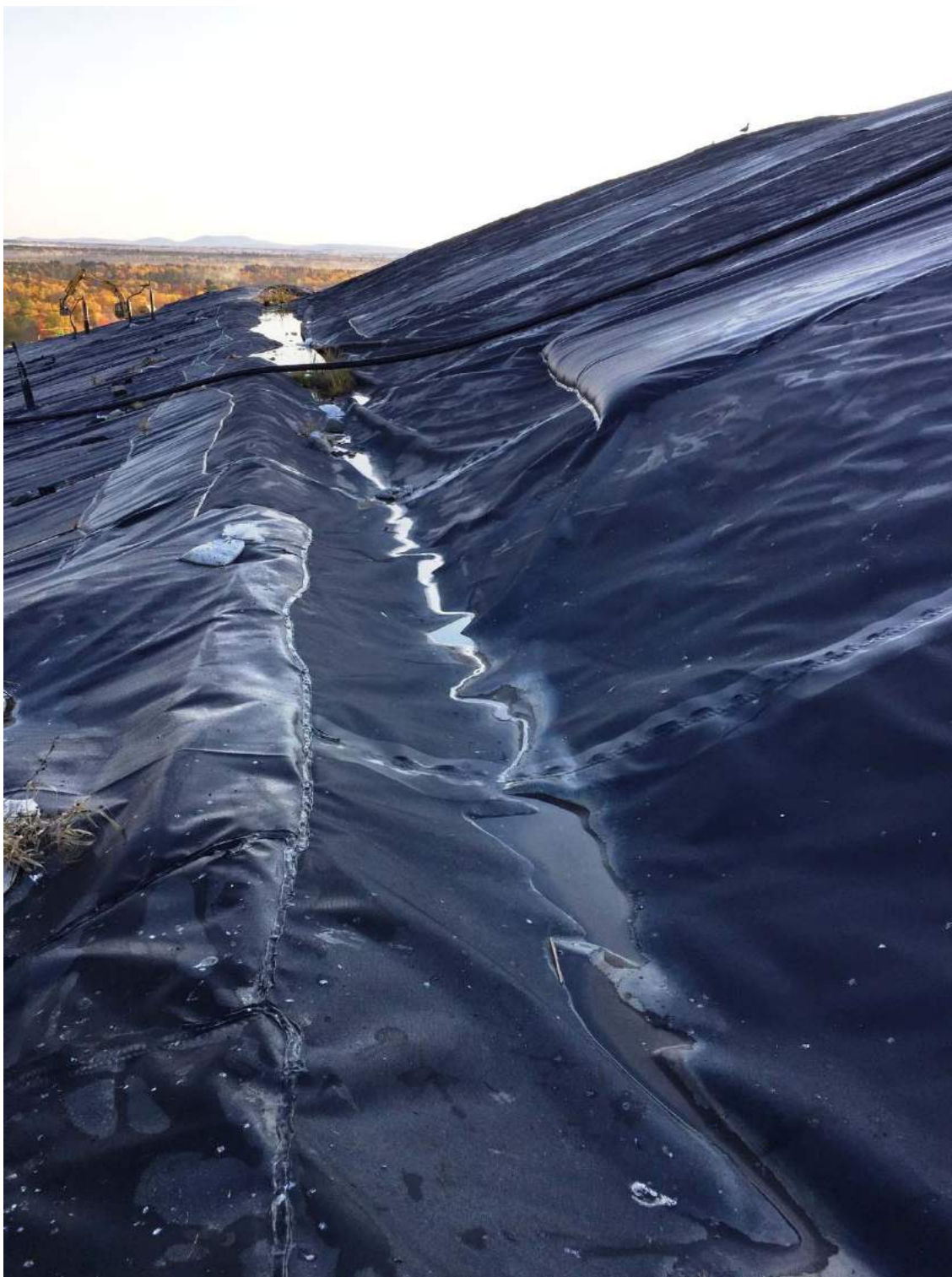
3. top northerneast slope looking northeast along surface water diversion & slope between Cell 3 & 7 (note: buldge in SICM)
