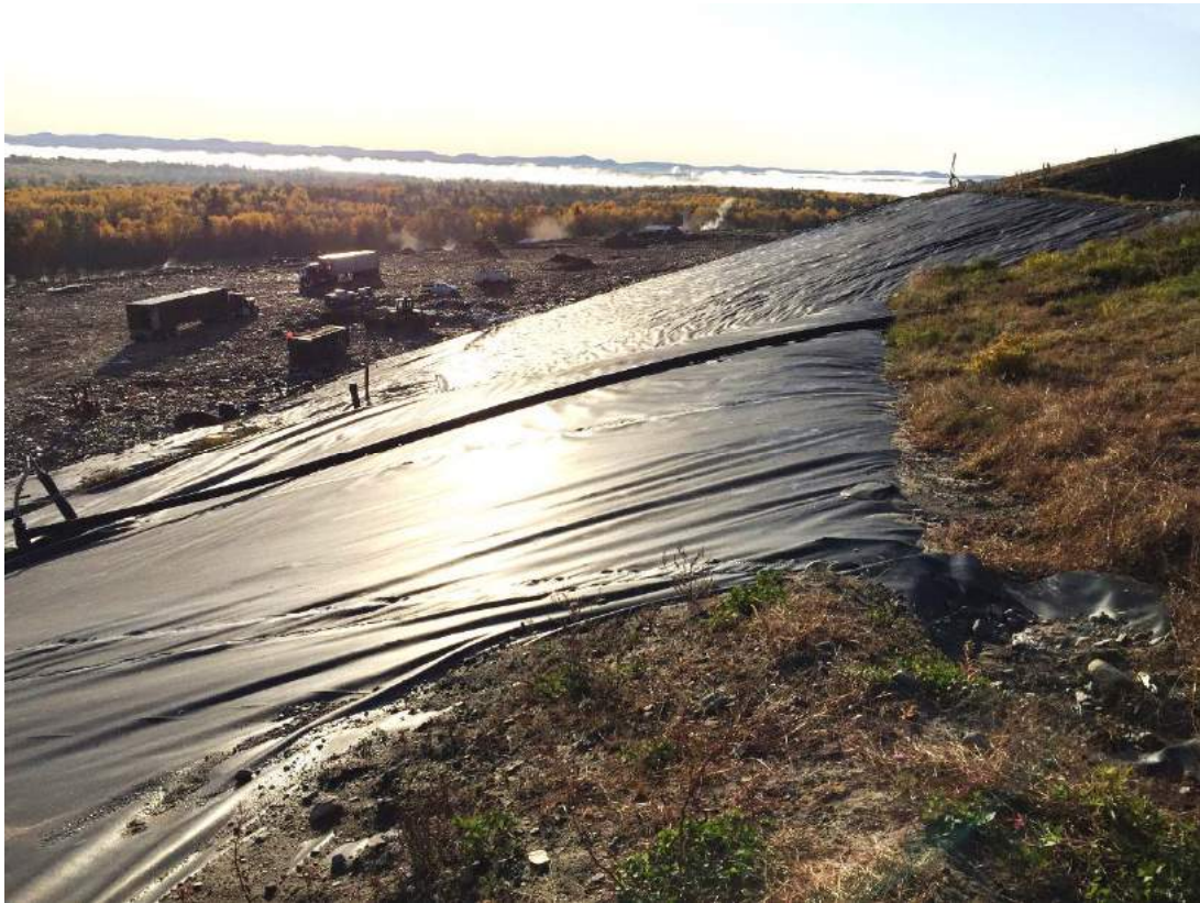
7. northeast corner of landfill Cell 7 looking southwesterly to northeast slope of Cell 9 & active Cell 11
