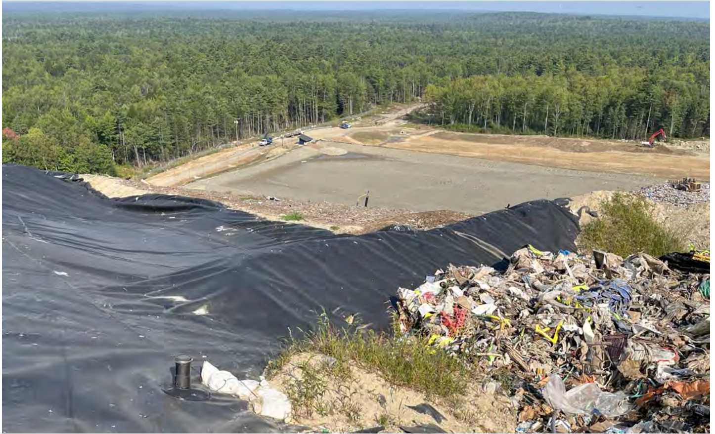
23. mid-height of southwest corner of Cells 1/2, looking down northwesterly slope of Cell 1 (note right: supplemental waste placed to bring the settled northern slope of Cells 1/2/3 back to final grade)
