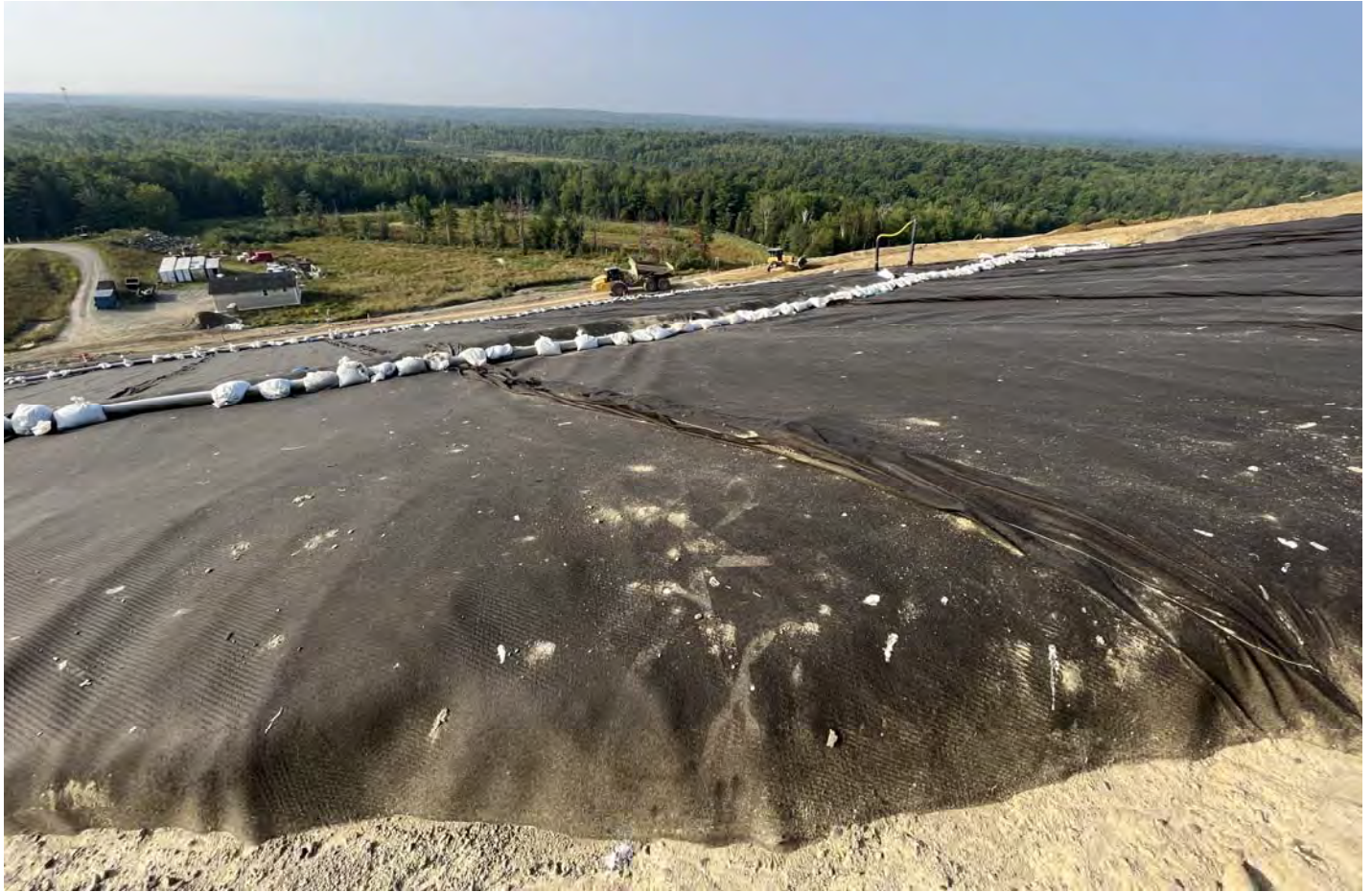
3. top of Cell 10 looking southerly down south slope of Cell 10
