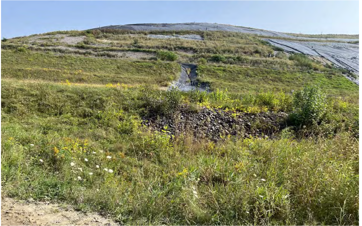
41. looking easterly up the slopes of Cells 1/2/3A
