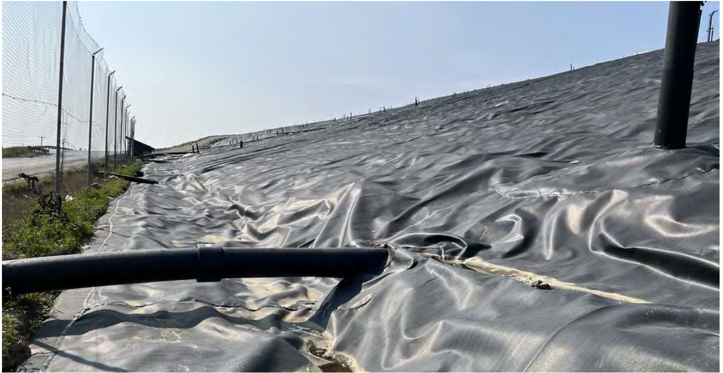
49. at the northeast corner of Cell 14 looking southeasterly at the toe of its easterly slope
