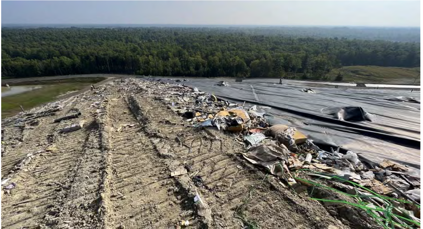
17. looking northeasterly down the north corner of Cell 14
