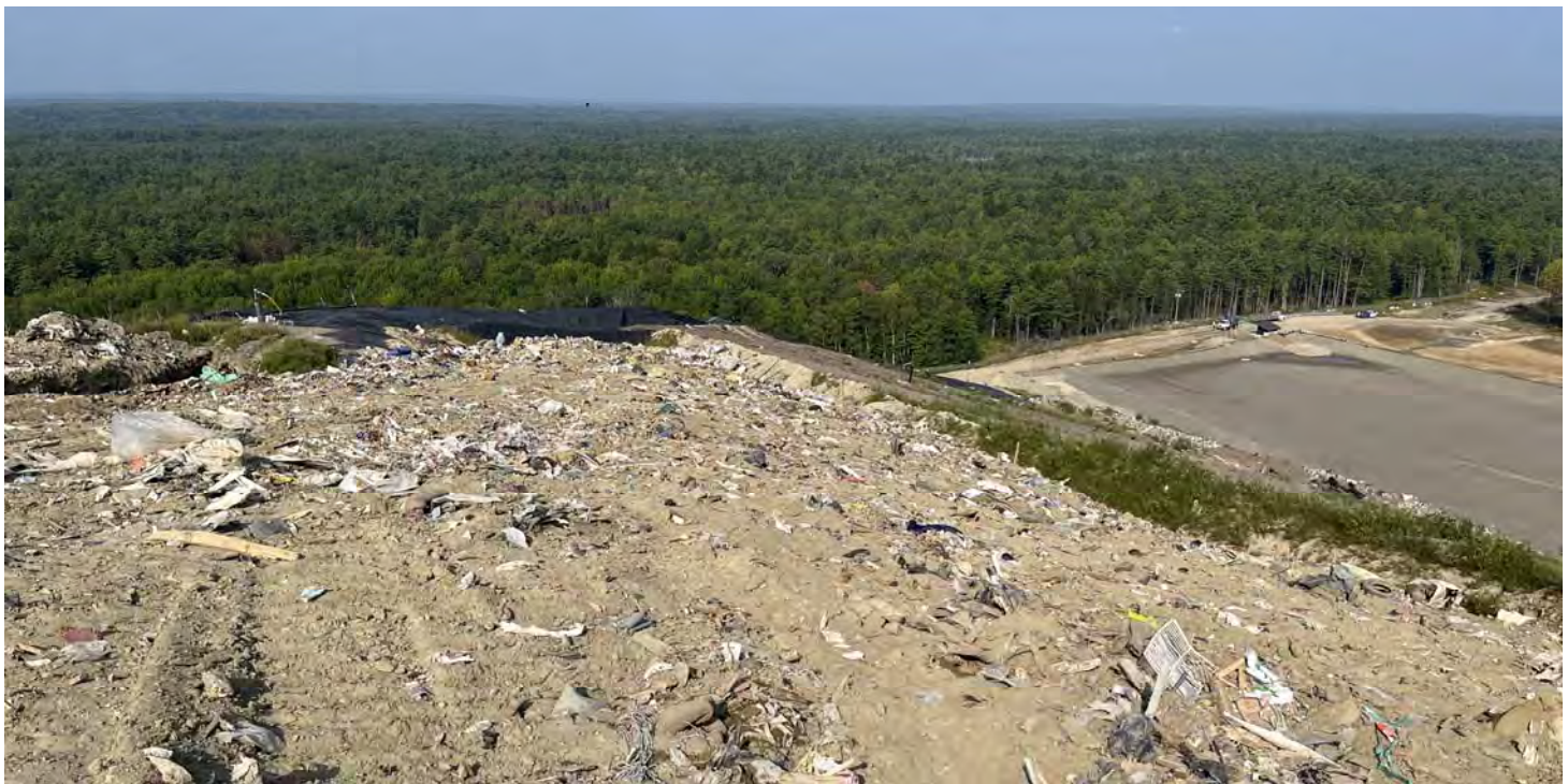
22. on top of the southwest corner of Cells 1/2, looking down towards the west ridge line
