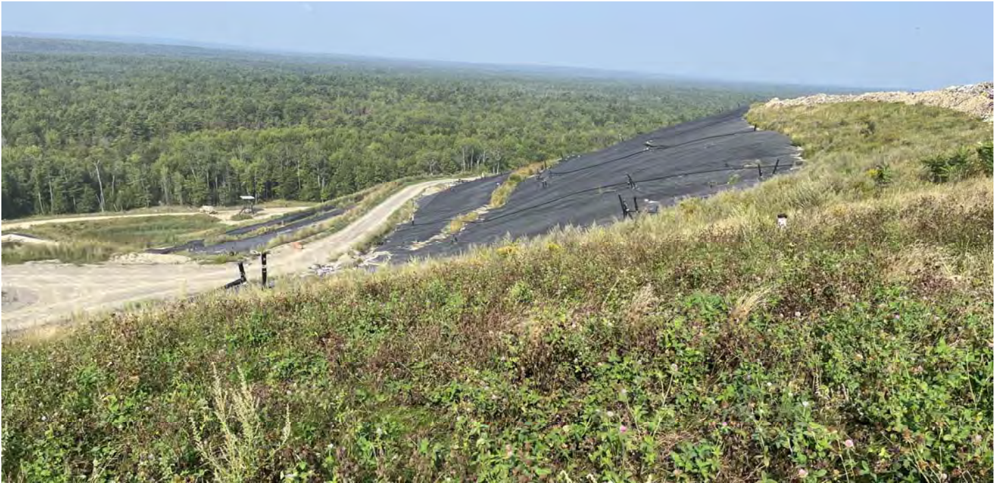
29. looking northwesterly towards upper slopes of Cells 4/3A/2/1
