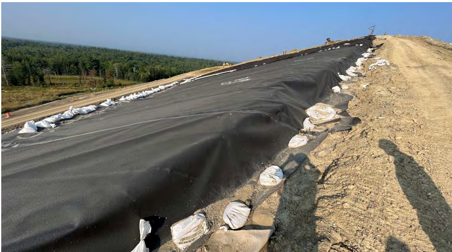
2. looking westerly toward closure activities on southern slope of Cell 10
