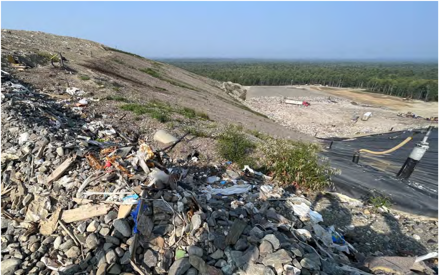
13. looking westerly along the northwest slope of Cells 1/2/3 and Cell 15 operations
