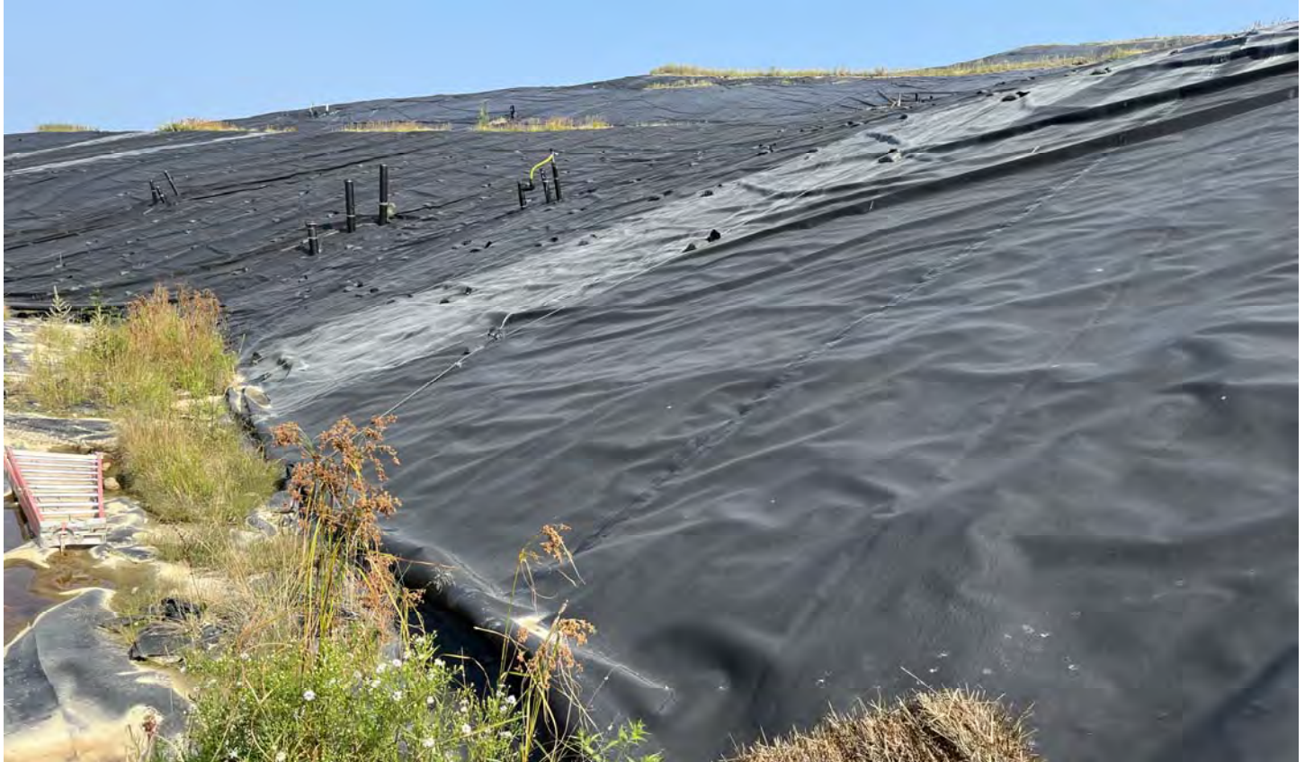
36. looking northerly at southerly slope of Cells 6/5/4
