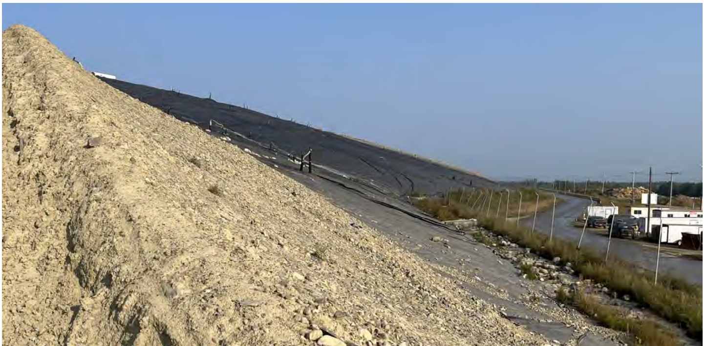
4. looking northwesterly along the easterly facing slope of Cells 10/11
