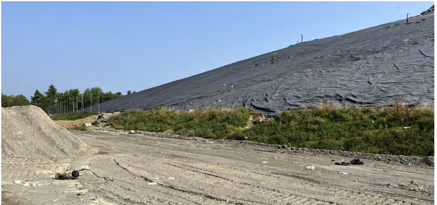
48. looking northerly at the northwesterly slope of Cell 14
