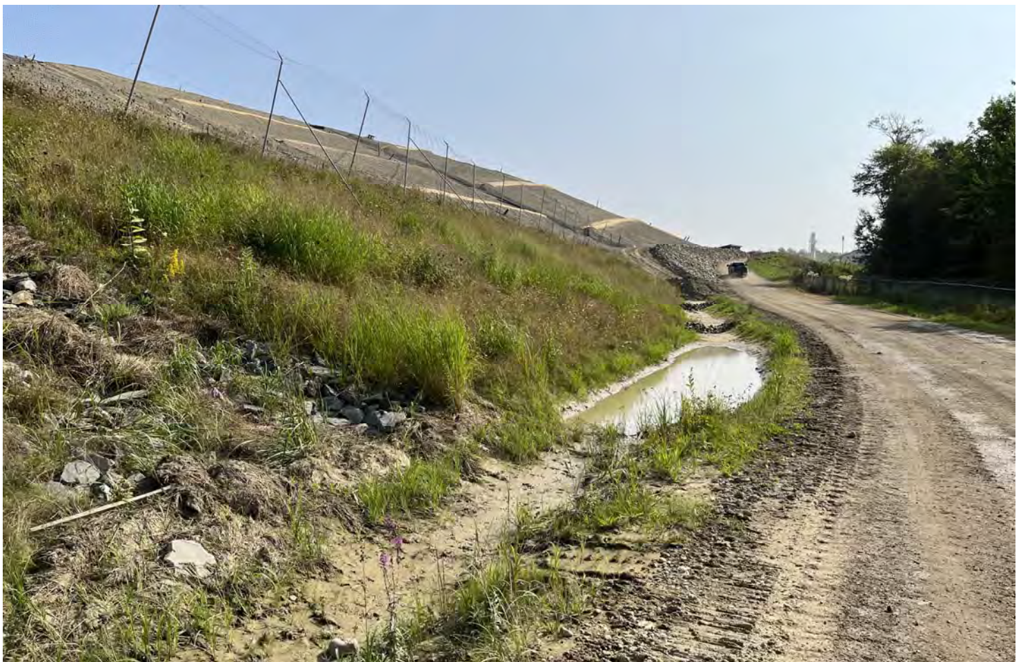
34. looking southeasterly along the southerly slope of Cell 8
