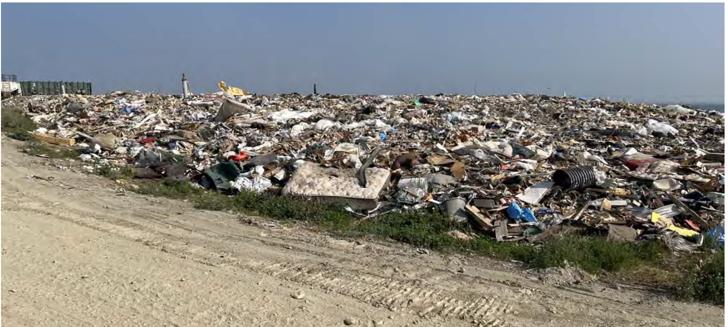
30. active grading waste placement on top of Cell 9
