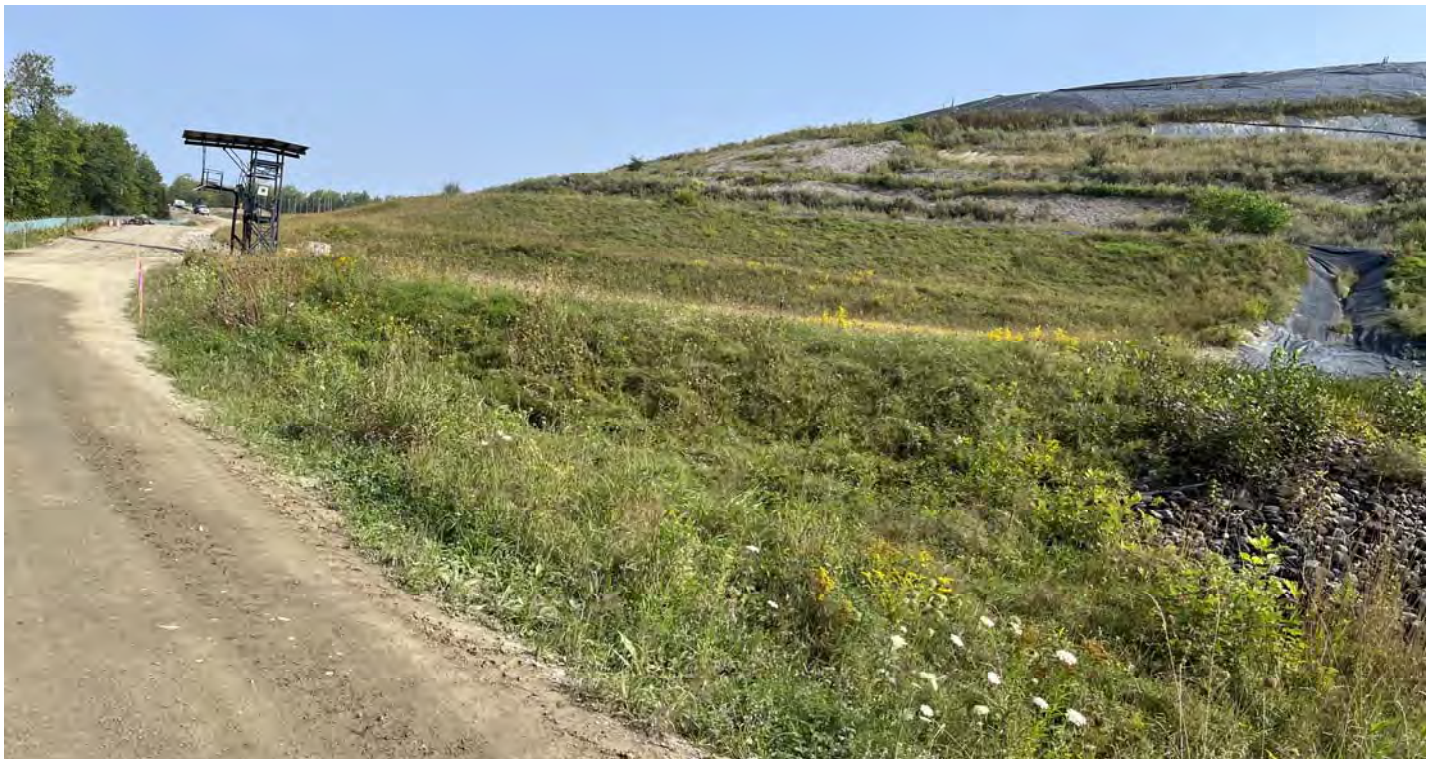
42. looking northerly along the slopes of Cells 1/2
