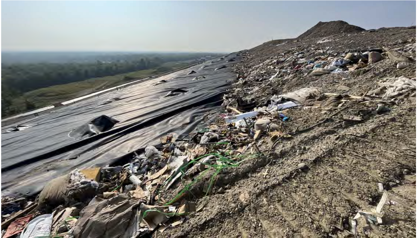
18. looking southeasterly along the geom-covered northeasterly slope of Cells 14/13
