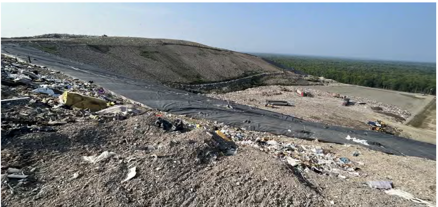
14. top of Cell 13/14 looking southwesterly down its SICM covered slope across to the northeasterly facing slope of Cells 1/2/3
