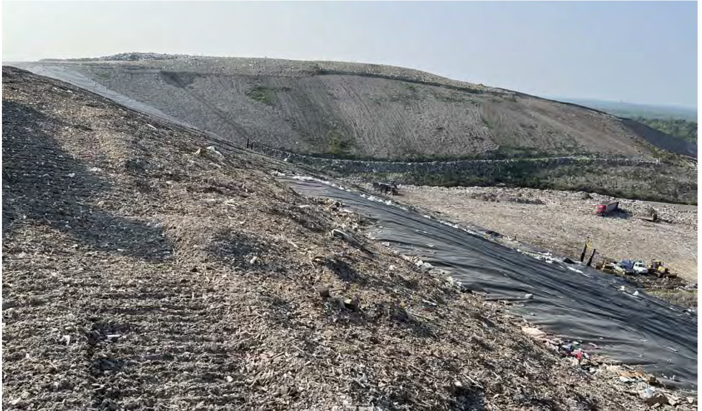
19. on the southwesterly slope of Cell 13/14 looking southeasterly towards the northwesterly slope of Cells 1/2/3
