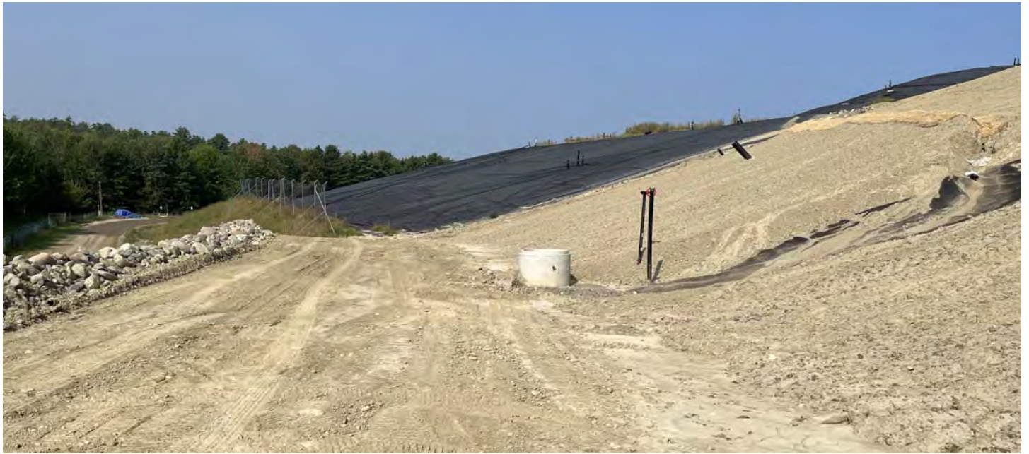
33. looking southwesterly along the southeasterly slope of Cell 10
