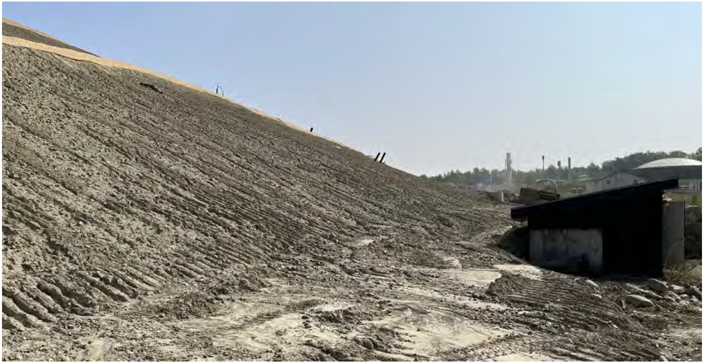
31. looking easterly along at the southeast landfill slope of Cell 10
