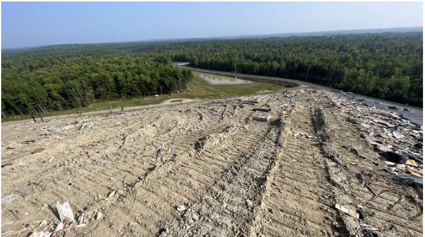
16. looking north-northeasterly down the north corner of Cell 14
