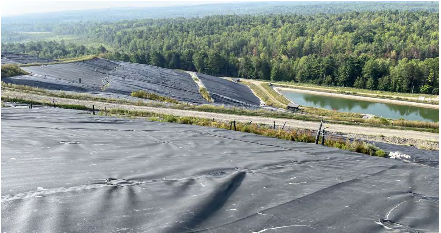
26. looking southeasterly along the lower slope of Cells 1/2/3A/4
