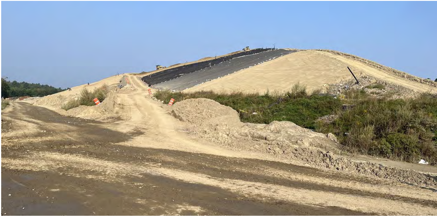
1. southeast corner of Cell 10 looking westerly along southern slope of Cell 10
