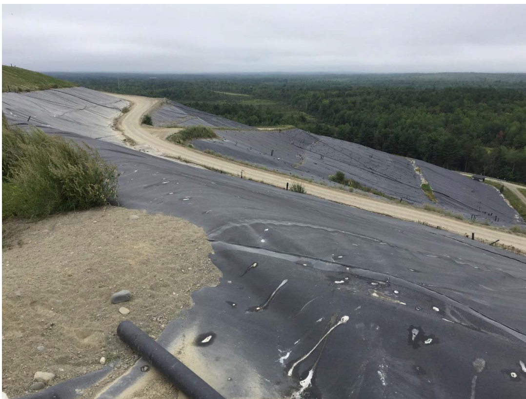
11. looking southeasterly across the upper southwesterly slope of Cells 4/5/6
