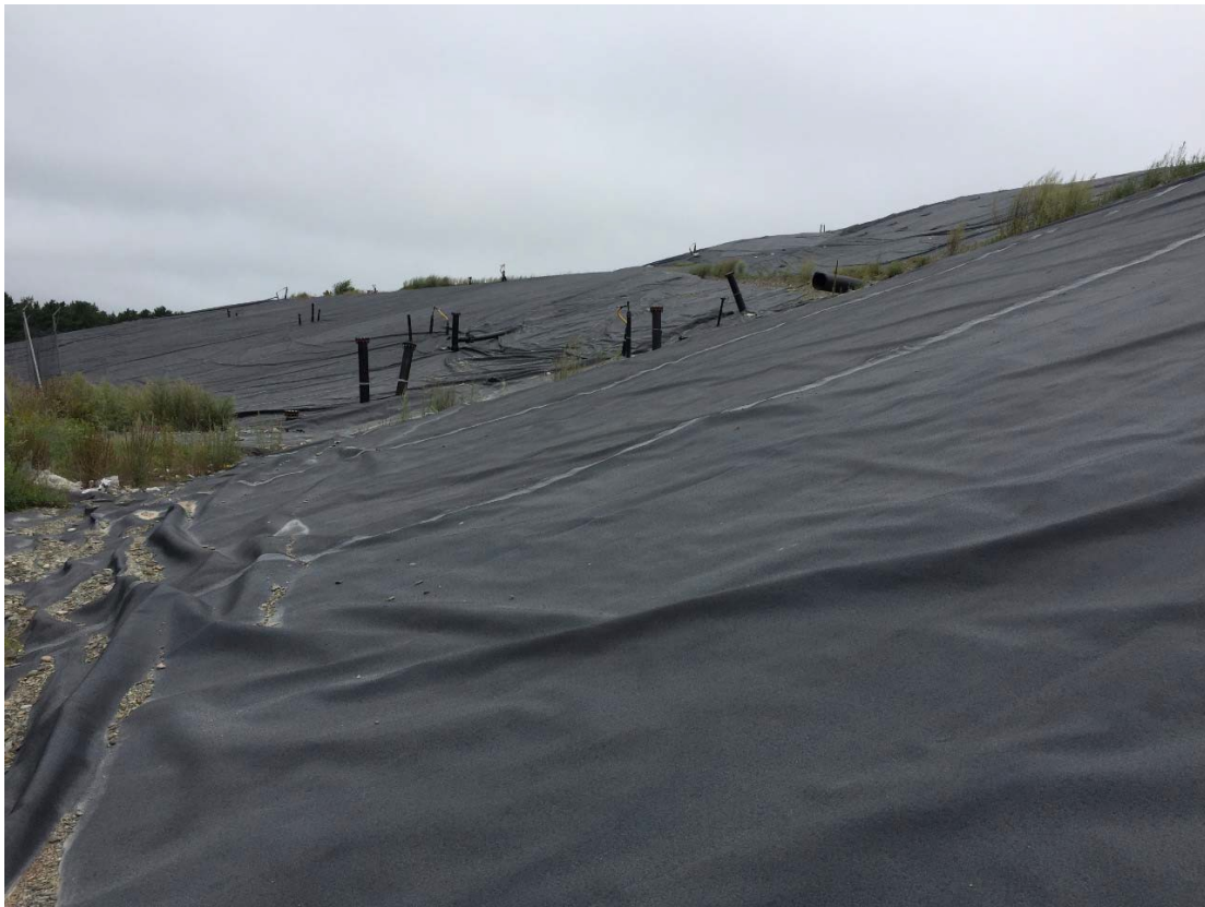
6. looking along the toe of the southeastern face of Cell 8 & Cell 10
