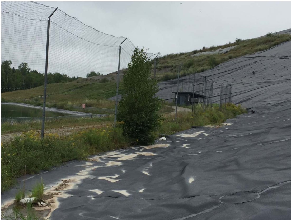
10. looking northwesterly along the westerly toe of Cells 1/2/4
