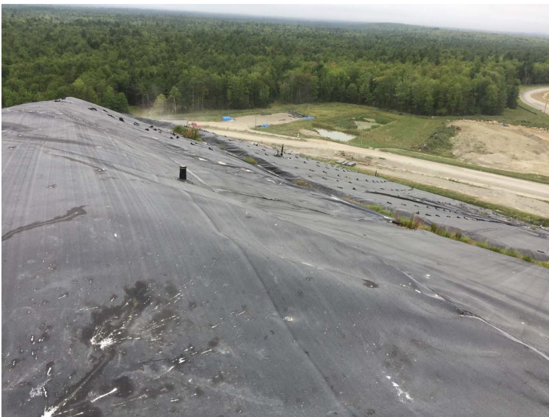
17. looking northwesterly along northern slope of Cells 1/2/3
