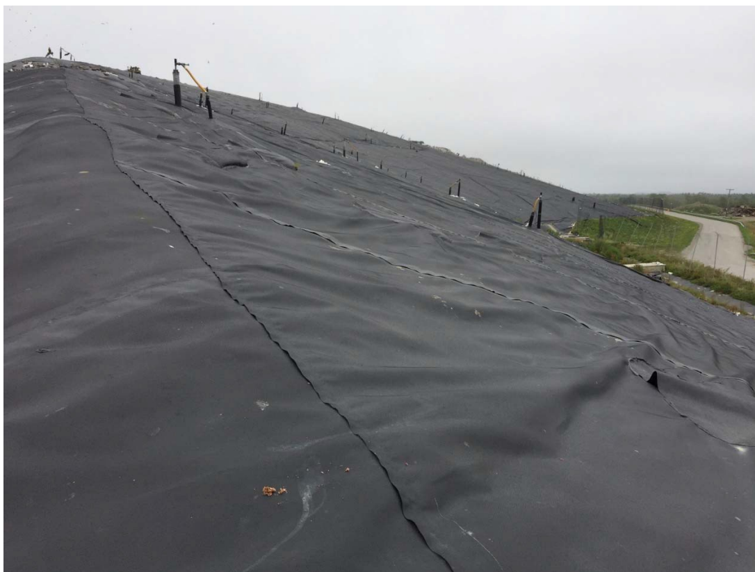
1. looking northwesterly along southwestern portion of the eastern slope of Cells 10/11
