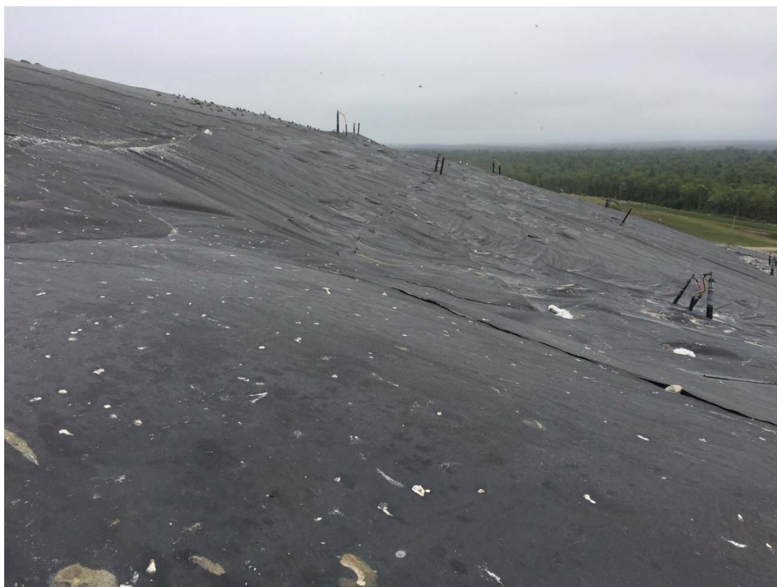
2. looking north along the central portion of Cells 10/11 eastern slope
