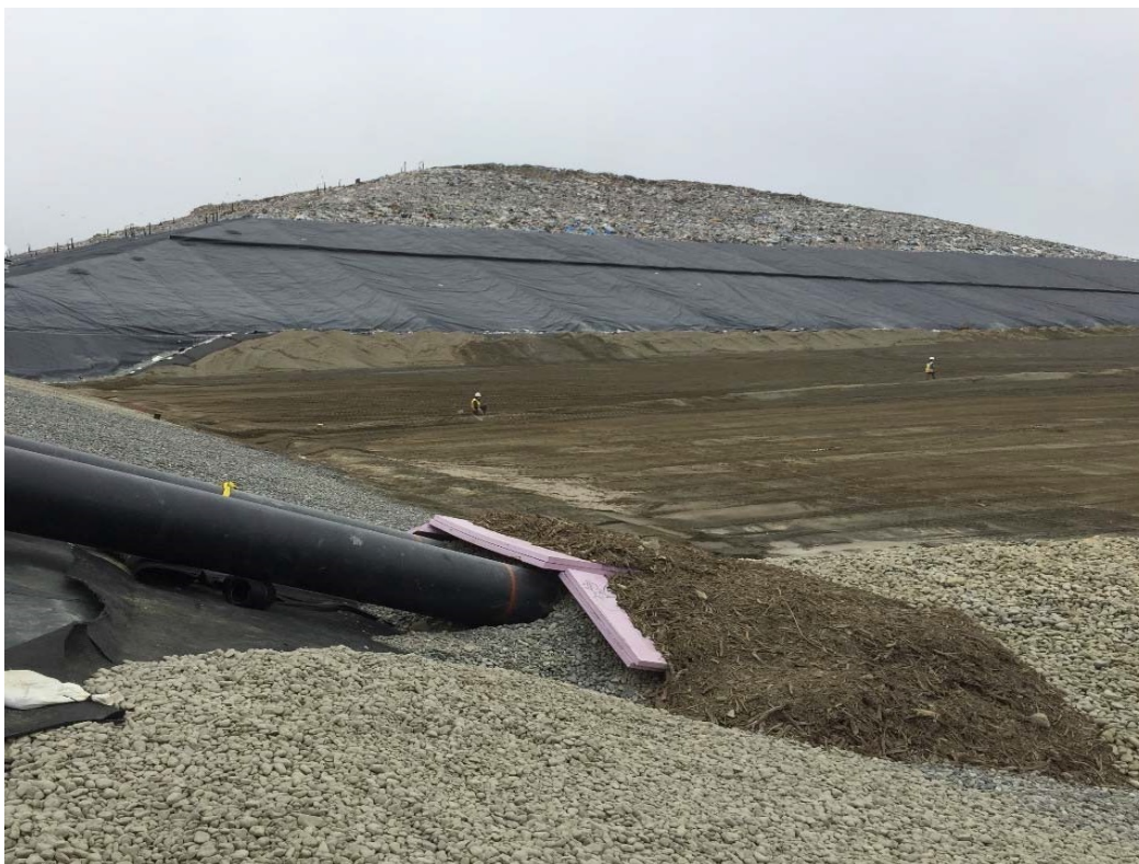
23. looking southeasterly along eastern portion of northern slope of Cell 12 (Cell 13 construction in the foreground)
