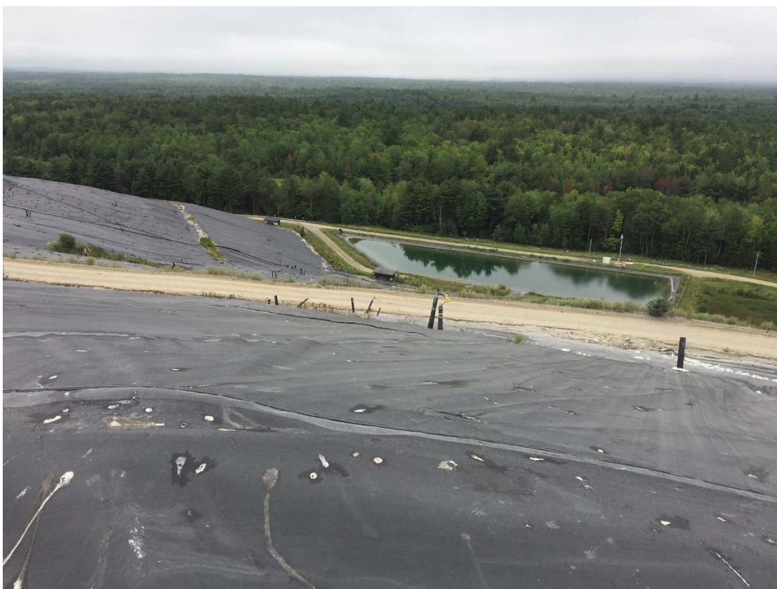
12. looking southwesterly down the westerly slope of Cells 4/5
