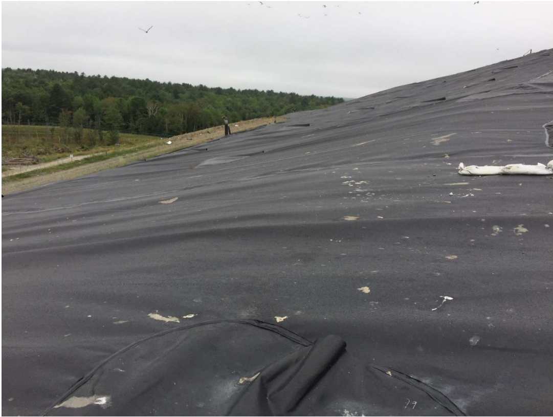
5. looking westerly across upper southeastern slope of Cell 10
