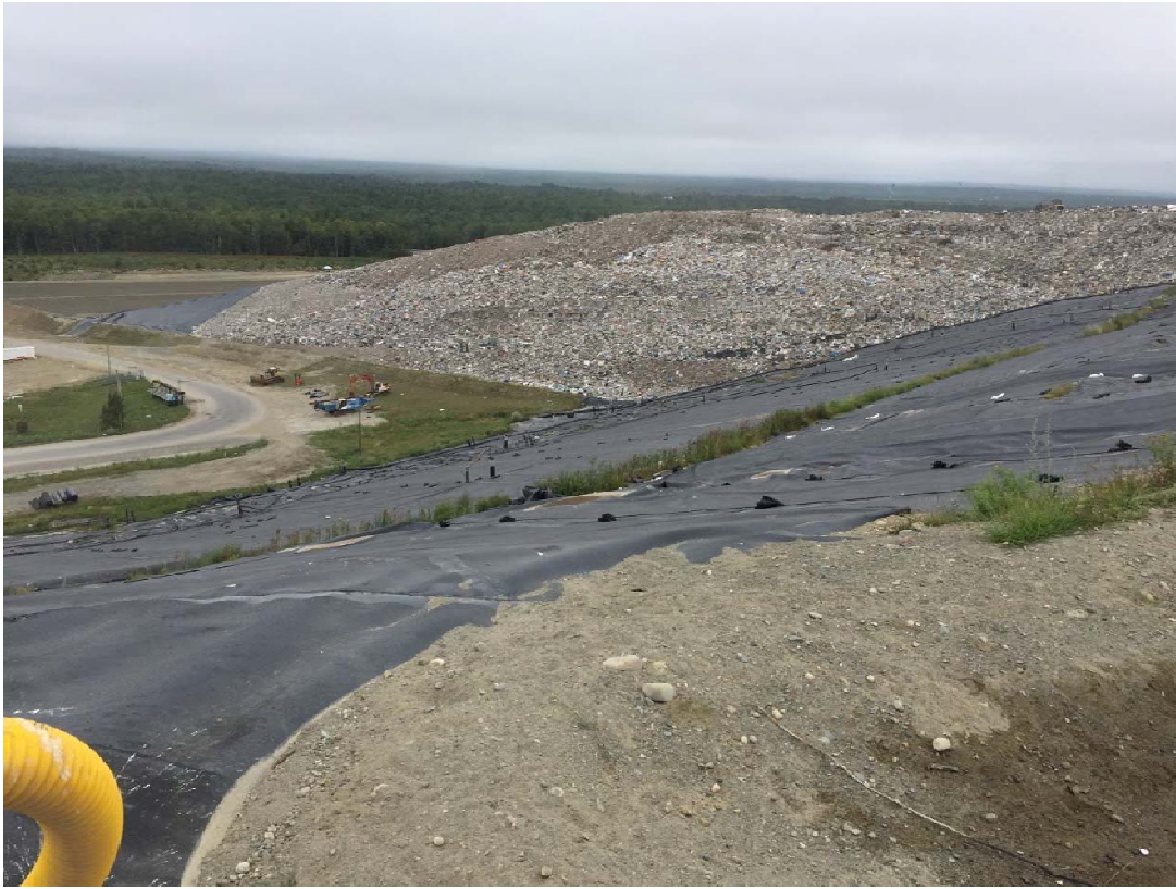
19. on the northern slope of Cell 7 looking northerly towards the active western slope of Cell 12
