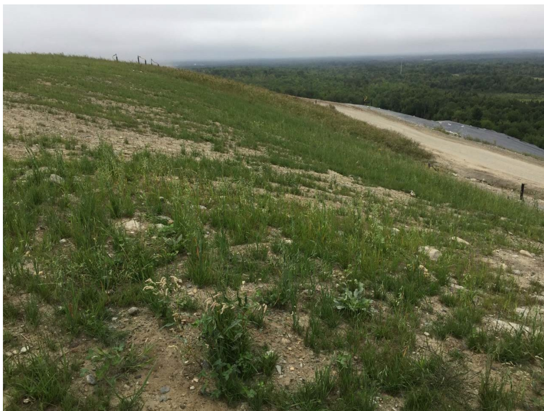
8. looking southerly along the upper portion of the southwestern slope of Cells 4/5
