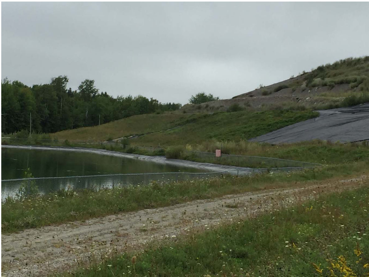
14. looking northwesterly along the lower portion of the southwestern slope of Cells 1/2/3/4
