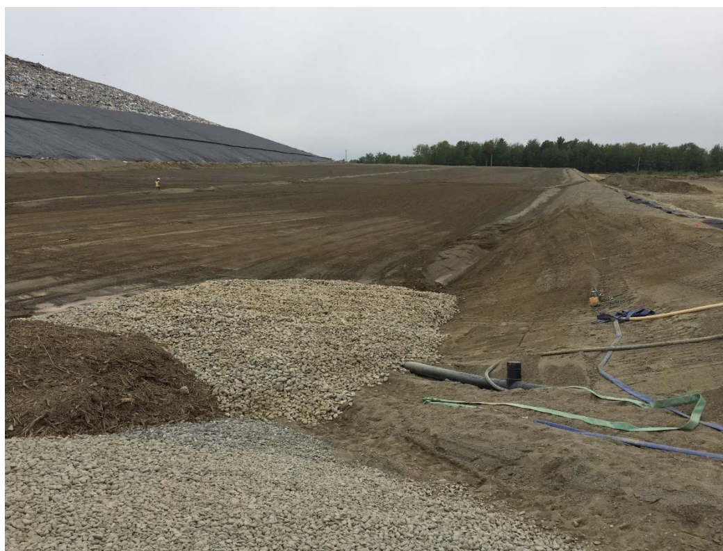
24. easterly across middle portion of northern slope of Cell 12 & Cell 13 construction
