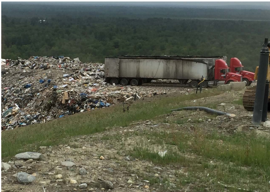
20. on the northern slope of Cell 7 looking northerly towards the active western slope of Cell 12
