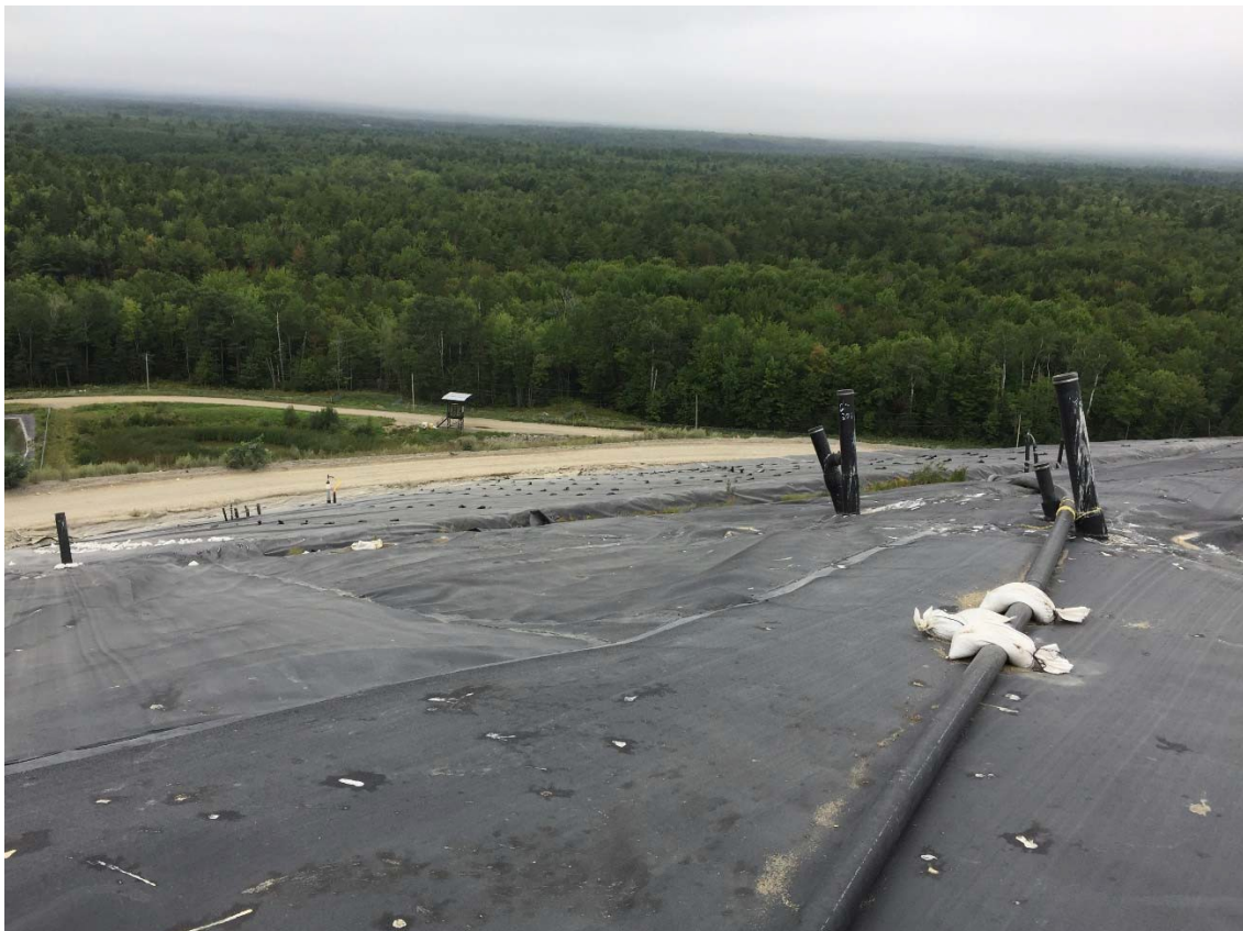
16. looking northwest down the westerly slope of Cells 2/3/4
