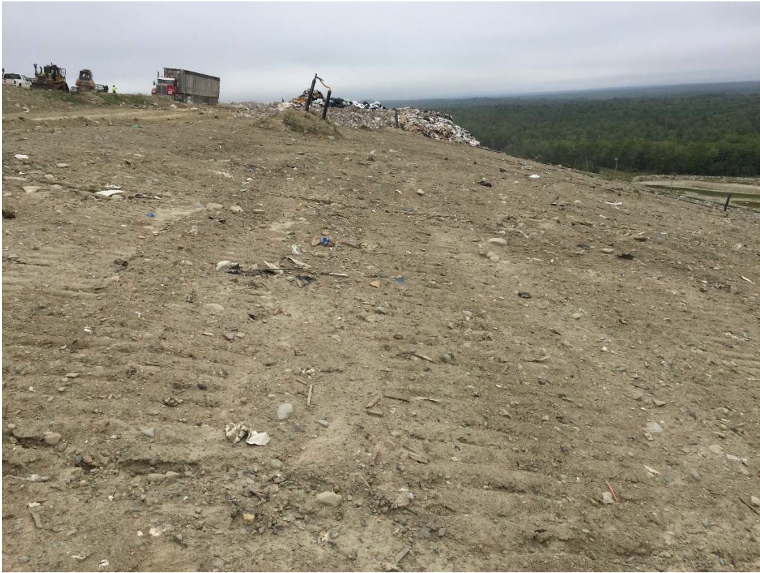
21. standing on the northeastern slope of Cell 11 looking northerly towards Cell 12 active area
