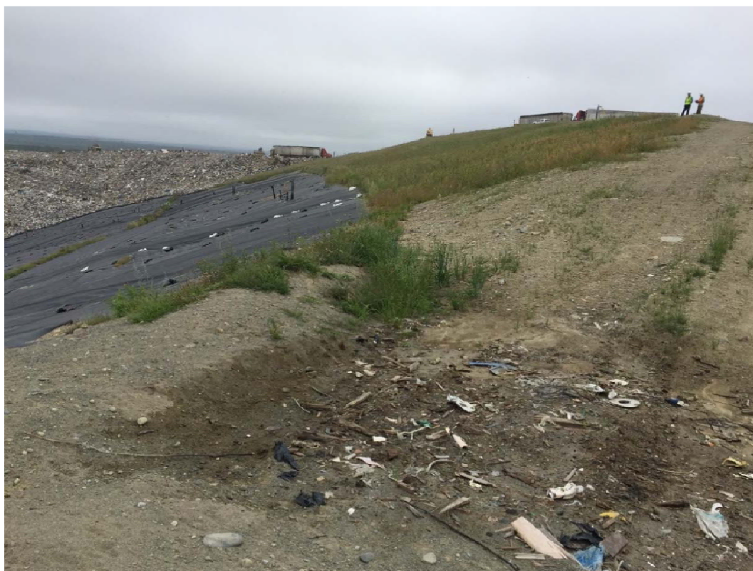
18. looking easterly along the northern slope of Cell 3 and the western slope of the active Cell 12
