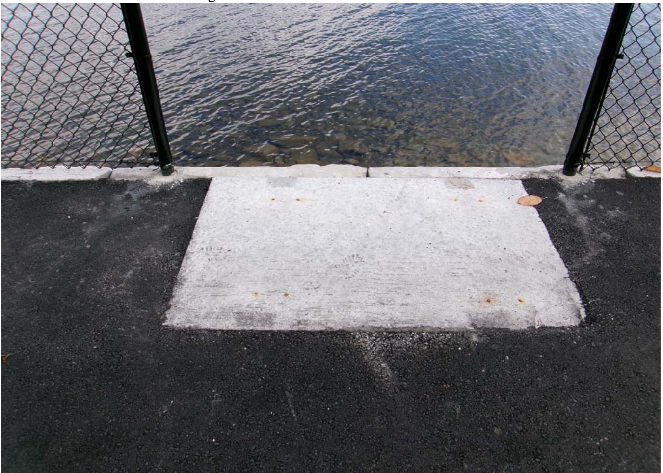
Photo #2 Fence Opening Concrete Wall Retaining Wall
