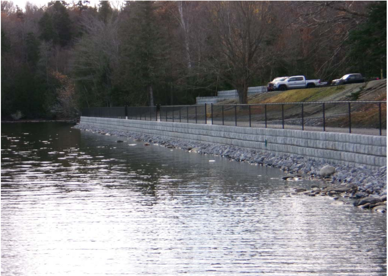
Photo #1 Concrete Box Retaining Wall
