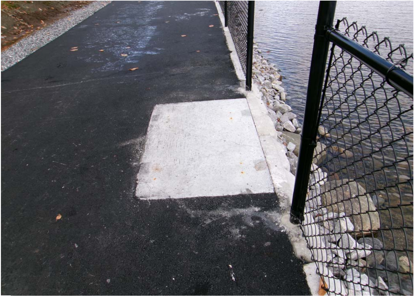
Photo #3 Fence Opening Concrete Wall Retaining Wall
