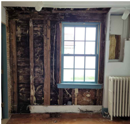
VIEW OF EAST WALL FRAMING IN FIRST FLOOR MUSEUM
