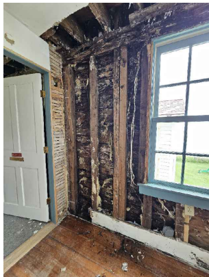
VIEW OF EAST WALL FRAMING IN FIRST FLOOR MUSEUM
