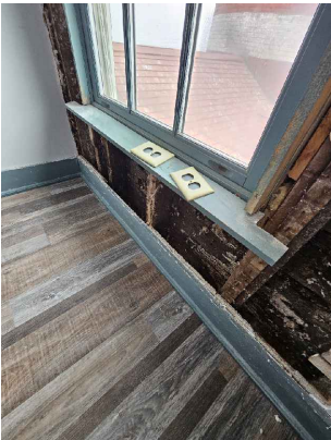
VIEW OF EAST WALL FRAMING IN SECOND FLOOR LIVING ROOM
