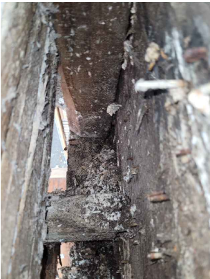
VIEW OF EAST WALL FRAMING AT SECOND FLOOR LIVING ROOM
