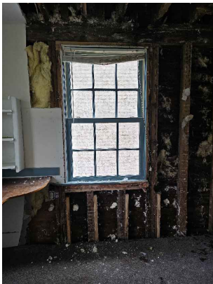
VIEW OF EAST WALL FRAMING IN FIRST FLOOR OFFICE
