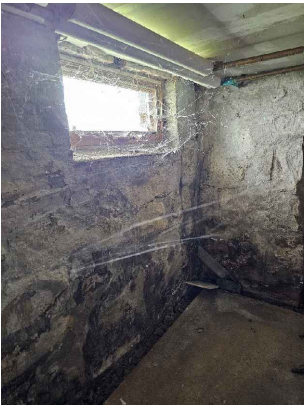
VIEW OF BASEMENT SHOWING WALL ADJACENT TO BULKHEAD ENTRANCE
