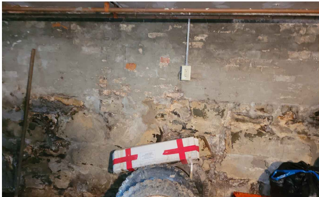
VIEW OF BASEMENT SHOWING EAST WALL OF MAIN PORTION OF RESIDENCE LOOKING EAST
