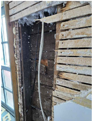
VIEW OF EAST WALL FRAMING IN SECOND FLOOR LIVING ROOM
