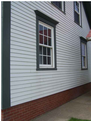
VIEW OF EAST SIDE OF KEEPER'S RESIDENCE SHOWING FIRST FLOOR WINDOWS AND FOUNDATION
