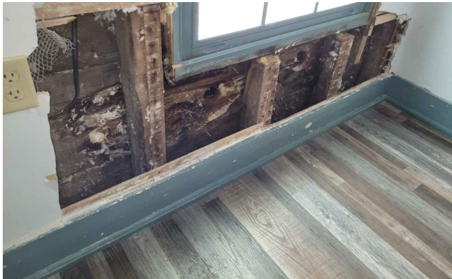
VIEW OF EAST WALL FRAMING IN SECOND FLOOR DINING ROOM
