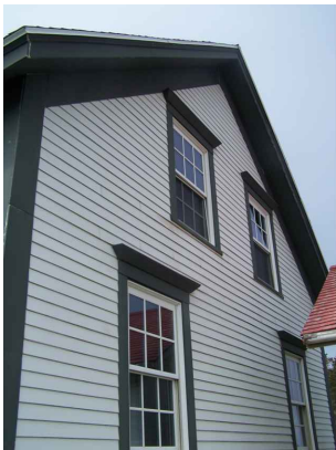
VIEW OF EAST SIDE OF KEEPER'S RESIDENCE SHOWING SECOND FLOOR WINDOWS
