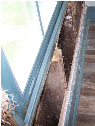
VIEW OF EAST WALL FRAMING IN SECOND FLOOR DINING ROOM
