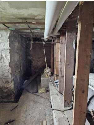
VIEW OF BASEMENT SHOWING SOUTHEAST CORNER OF BUILDING
