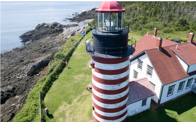
VIEW OF EAST SIDE OF KEEPER'S RESIDENCE AND SITE SHOWING PROXIMITY TO OCEAN
