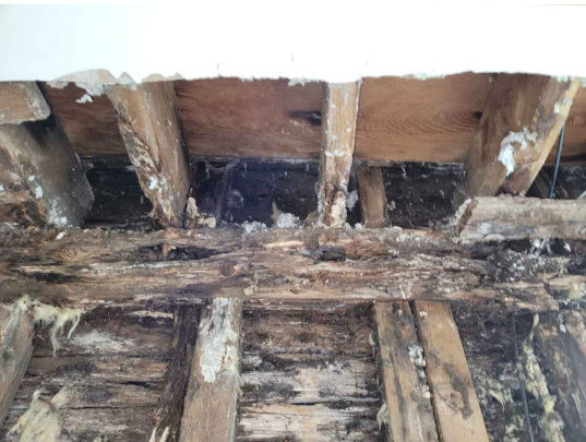
VIEW OF EAST WALL IN FIRST FLOOR MUSEUM SHOWING WALL AND CEILING FRAMING
