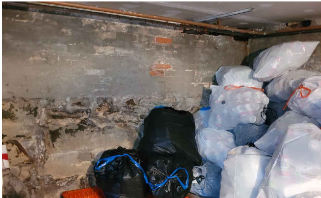
VIEW OF BASEMENT SHOWING EAST WALL OF MAIN PORTION OF RESIDENCE LOOKING TOWARDS SOUTHEAST CORNER
