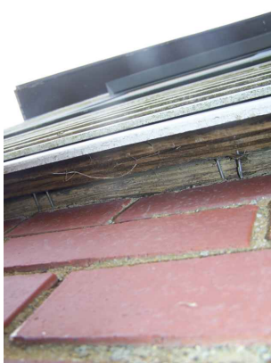
VIEW OF EAST SIDE OF KEEPER'S RESIDENCE SHOWING CURRENT SHEATHING AND SIDING ASSEMBLY
