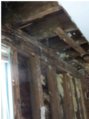
VIEW OF EAST WALL IN FIRST FLOOR OFFICE SHOWING WALL AND CEILING FRAMING
