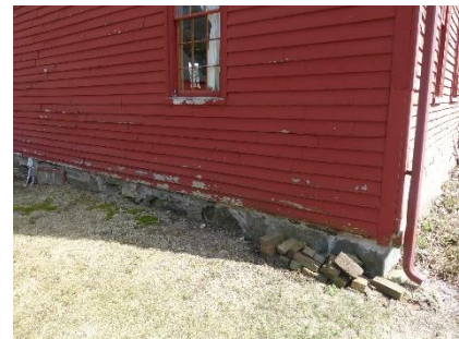
Fieldstone foundation at west wall
