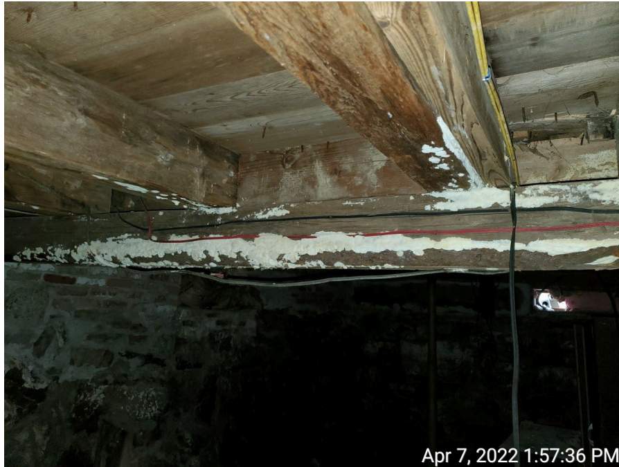
View of "wet rot" fungi for wood framing in basement area.
