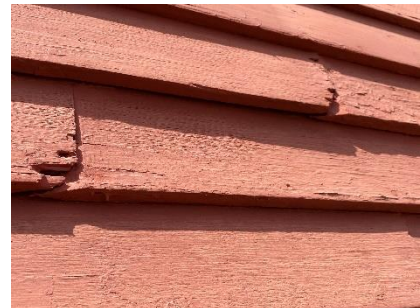
Skived joints at clapboards
