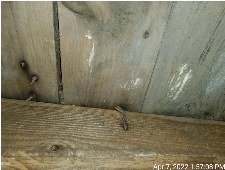
Apr 7, 2022 1:57:03 PM View of "wet rot" fungi for wood framing in basement area.
