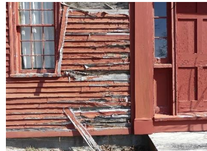
Skived joints at clapboards
