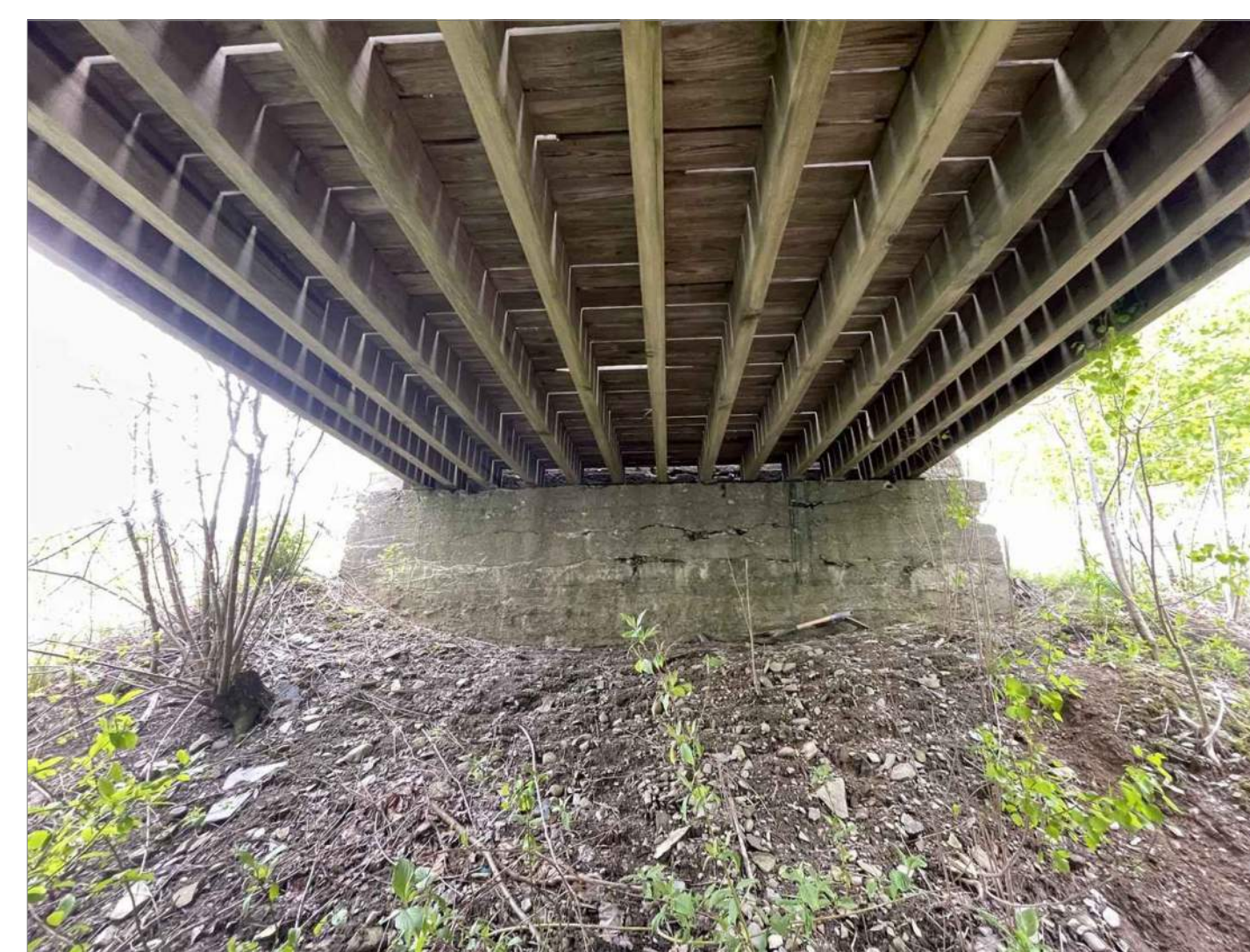
C2 IMAGE OF UNDERSIDE OF BRIDGE
