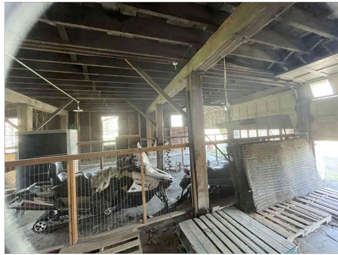
A3 IMAGE OF LOWER LEVEL WEST BAY
