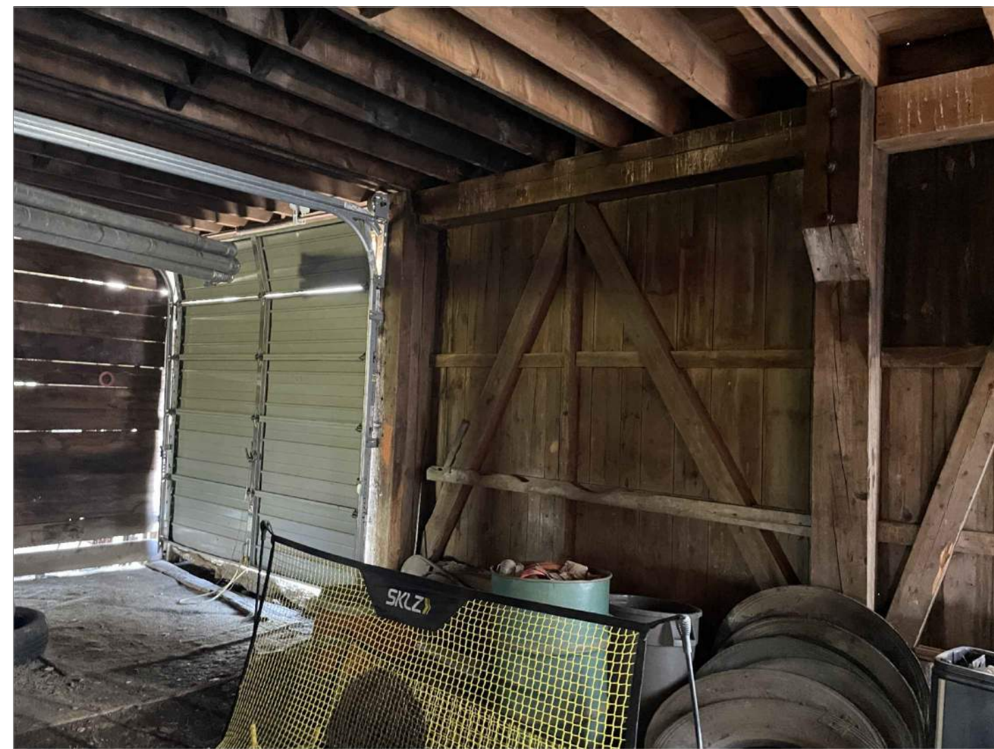
A2 IMAGE OF LOWER LEVEL MIDDLE BAY
