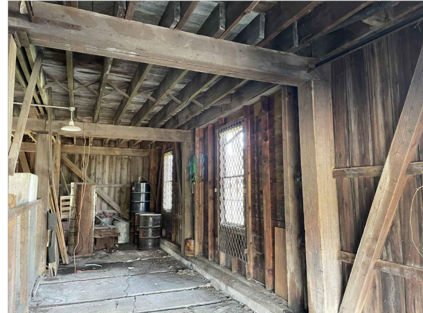
B3 IMAGE OF LOWER LEVEL WEST WALL
