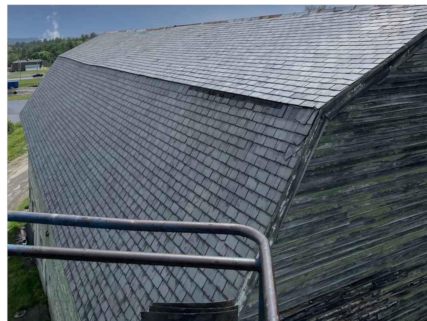
A1 IMAGE OF NORTHEAST ROOF CONDITION
