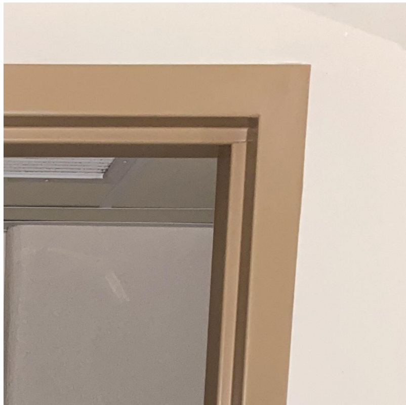
EXISTING TYPICAL HM DOOR FRAME
