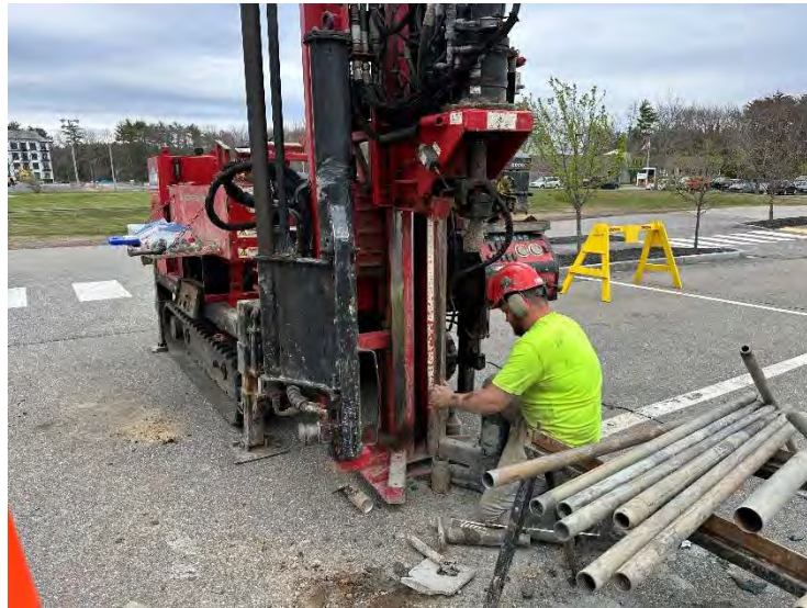
Performance of Field Vane at Test Boring B-2, Facing East
