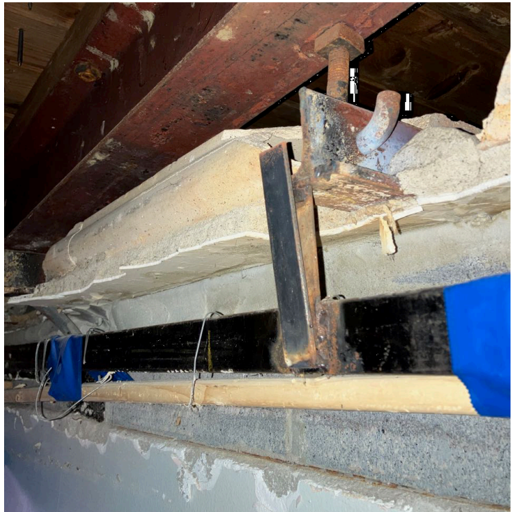
ROOM 155 SUSPENDED TERRA COTTA CEILING TO BE REMOVED SO THAT STEEL AND DECK ABOVE CAN BE FIREPROOFED
