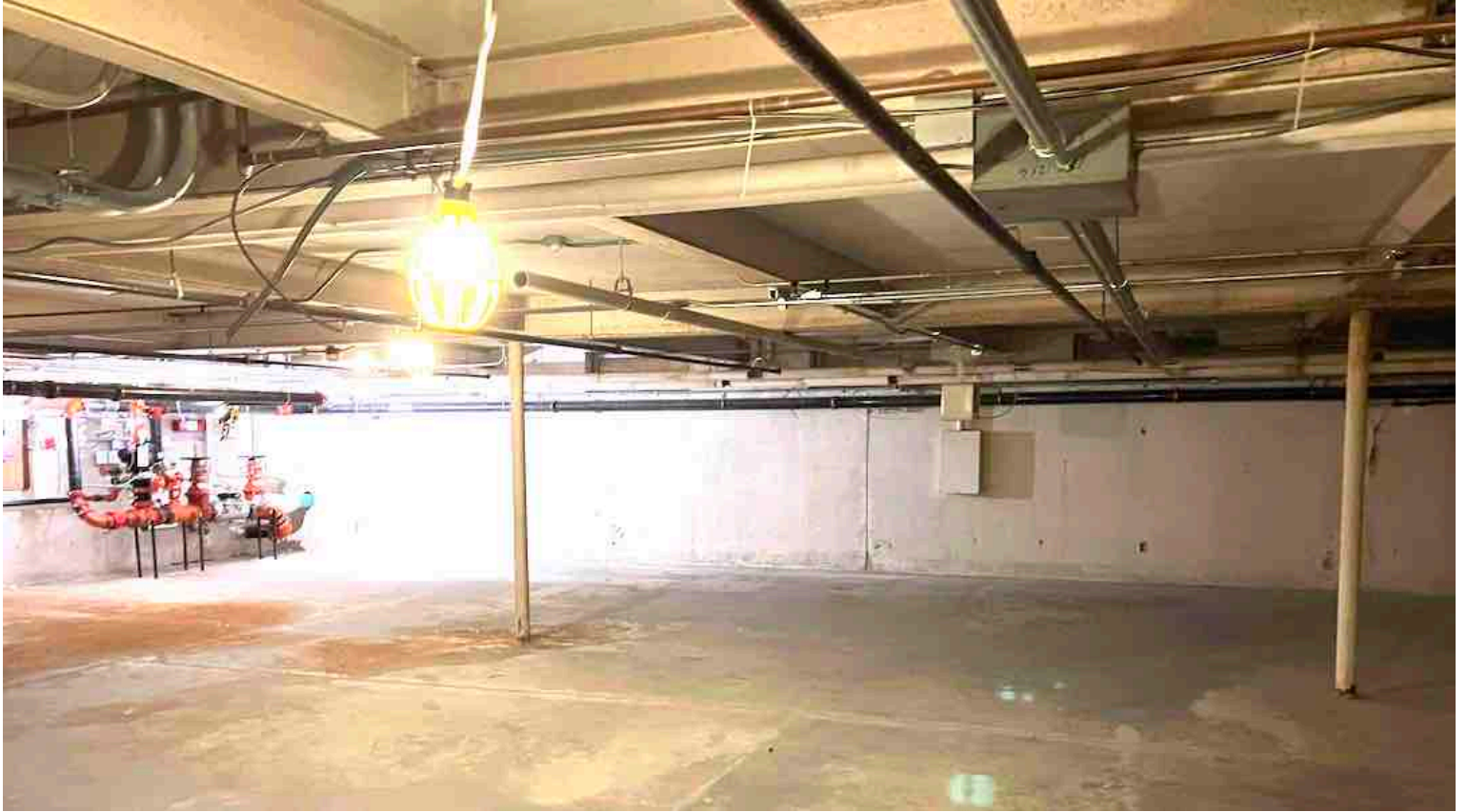
1957 STEEL FRAMING WITH FLAT CONC SLAB
