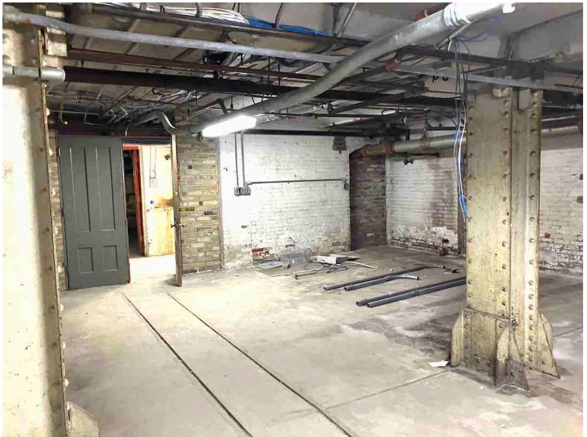
BASEMENT BUILT UP COLUMN : NORTHWEST
