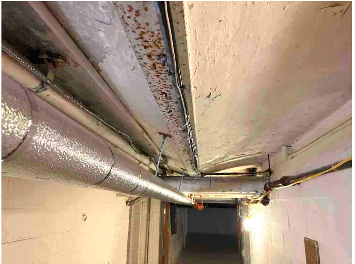
BASEMENT BRICK ARCH STEEL EXPOSED BOTTOM FLANGE
