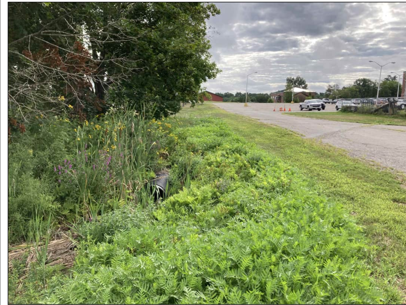
PHOTO 4 - 27"Ø HDPE STORM DRAIN OUTLET
