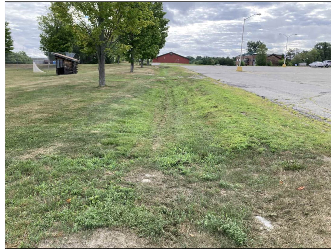
PHOTO 3 - GRASS SWALE AND CULVERTS TO BE REPLACED
