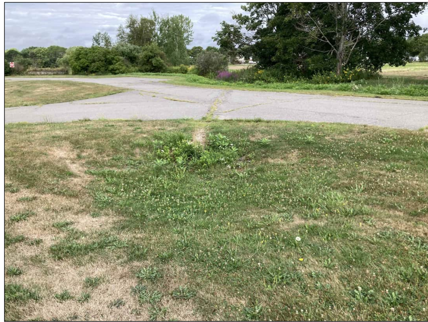
PHOTO 6 - 18"Ø CULVERT TO BE REPLACED
