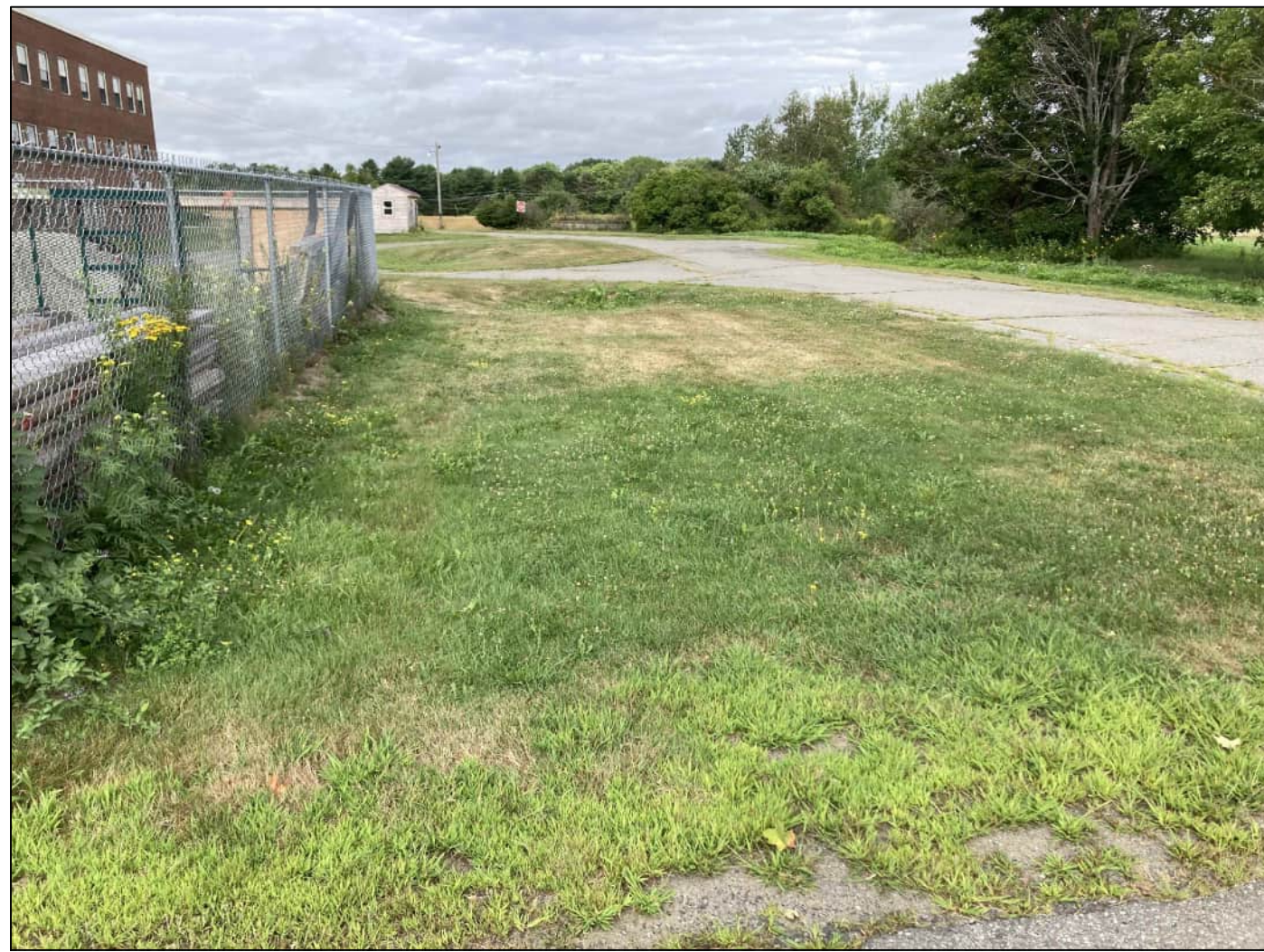
PHOTO 5 - INLET AREA TO 18"Ø CULVERT TO BE REPLACED
