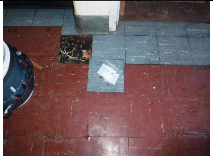
Photo 10 (12-16-2021): ACM 9-inch floor tile (NO-1-04) and PACM mastic and 9-inch floor tile located in North Wing – Section III.
