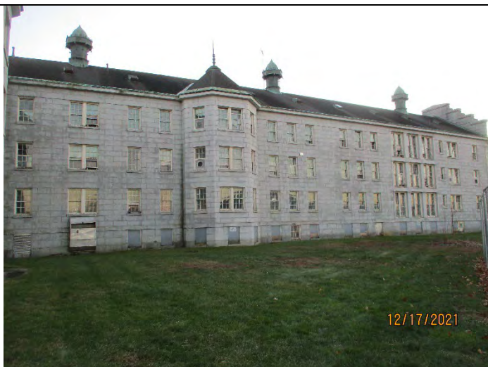
Photo 5 (12-17-2021): North Wing – Section II.
