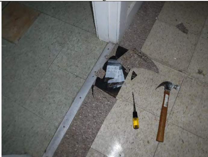
Photo 3 (12-16-2021): ACM mastic (NO-3-14) associated with multiple 12-inch floor tiles located throughout North Wing – Section II and III.
