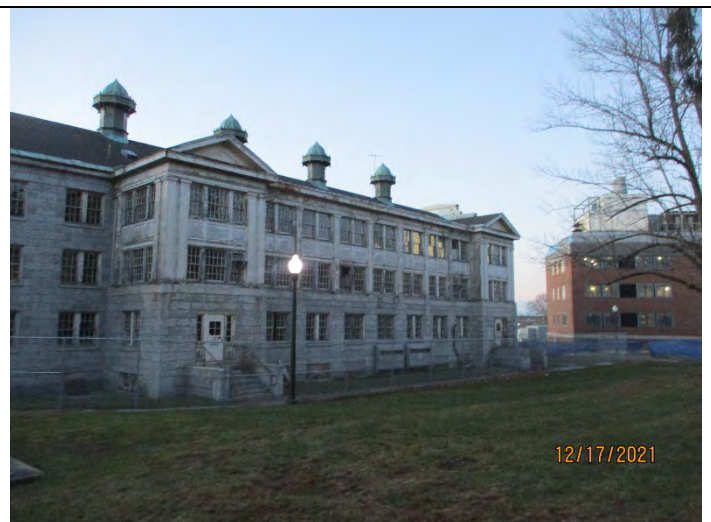
Photo 6 (12-17-2021): North Wing – Section III.
