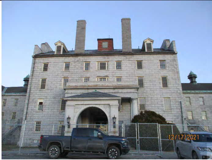
Photo 1 (12-17-2021): Front of Site building, Administrative building/area. South wing Section I on right, North wing Section I on left.
