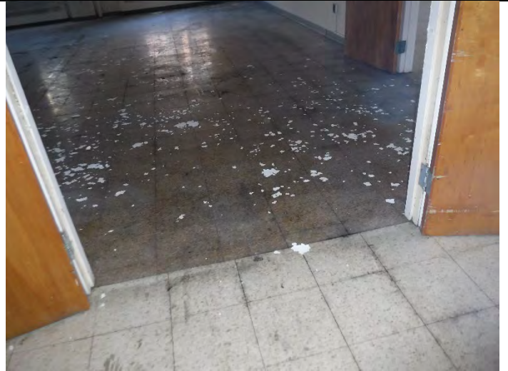
Photo 2 (12-17-2021): ACM 12-inch floor tiles (NO-3-30) located in select areas/room of South Wing – Sections II and III
