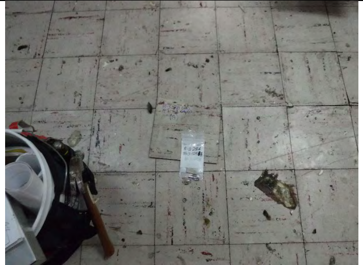
Photo 8 (12-16-2021): PACM 9-inch floor tile (NO-3-28) and associated ACM mastic (NO-3-29) located in North Wing – Section III.
