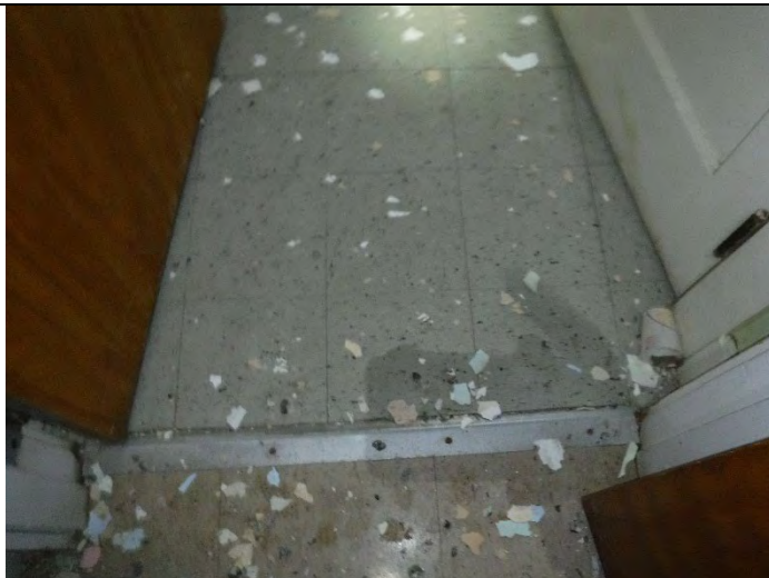
Photo 5 (12-16-2021): ACM 9-inch floor tile (NO-3-19) located in North Wing – Section II.
