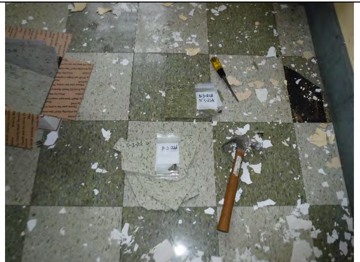
Photo 6 (12-16-2021): ACM 12-inch floor tile (NO-3-21) and ACM mastic (NO-3-26) located in various rooms throughout North Wing – Sections II and III.
