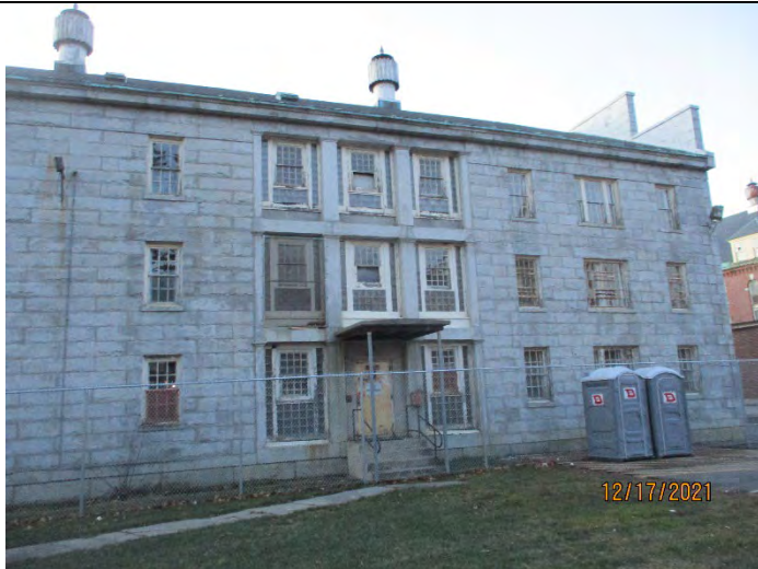
Photo 3 (12-17-2021): Portion of South Wing – Section III.
