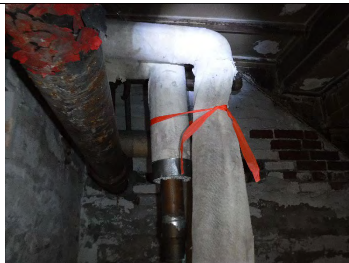
Photo 3 (12-17-2021): Location of positive ACM samples B-02A and B-03A
