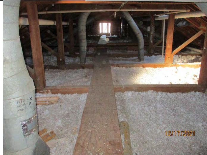
Photo 1 (12-17-2021): Representative photo of attic area.
