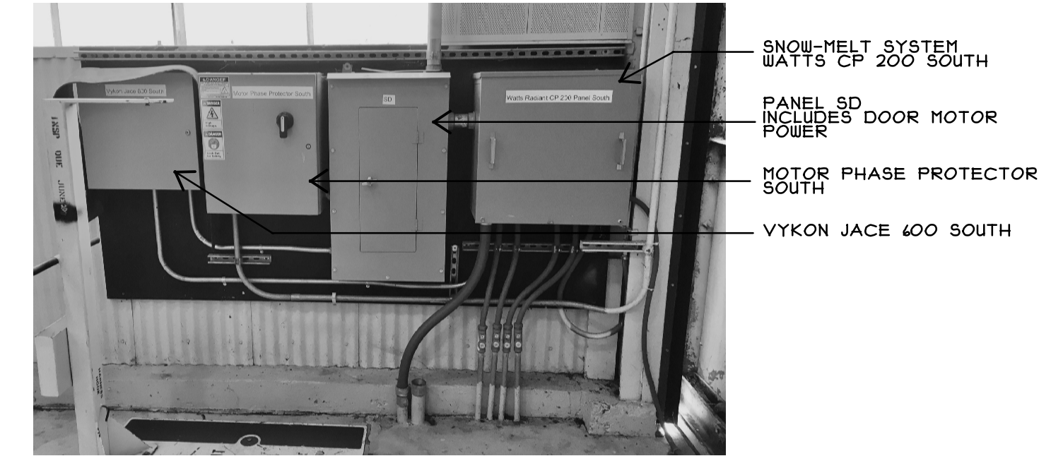
B-101 EXG ELCTRICAL AND CONTROL PANELS SOUTH WALL
