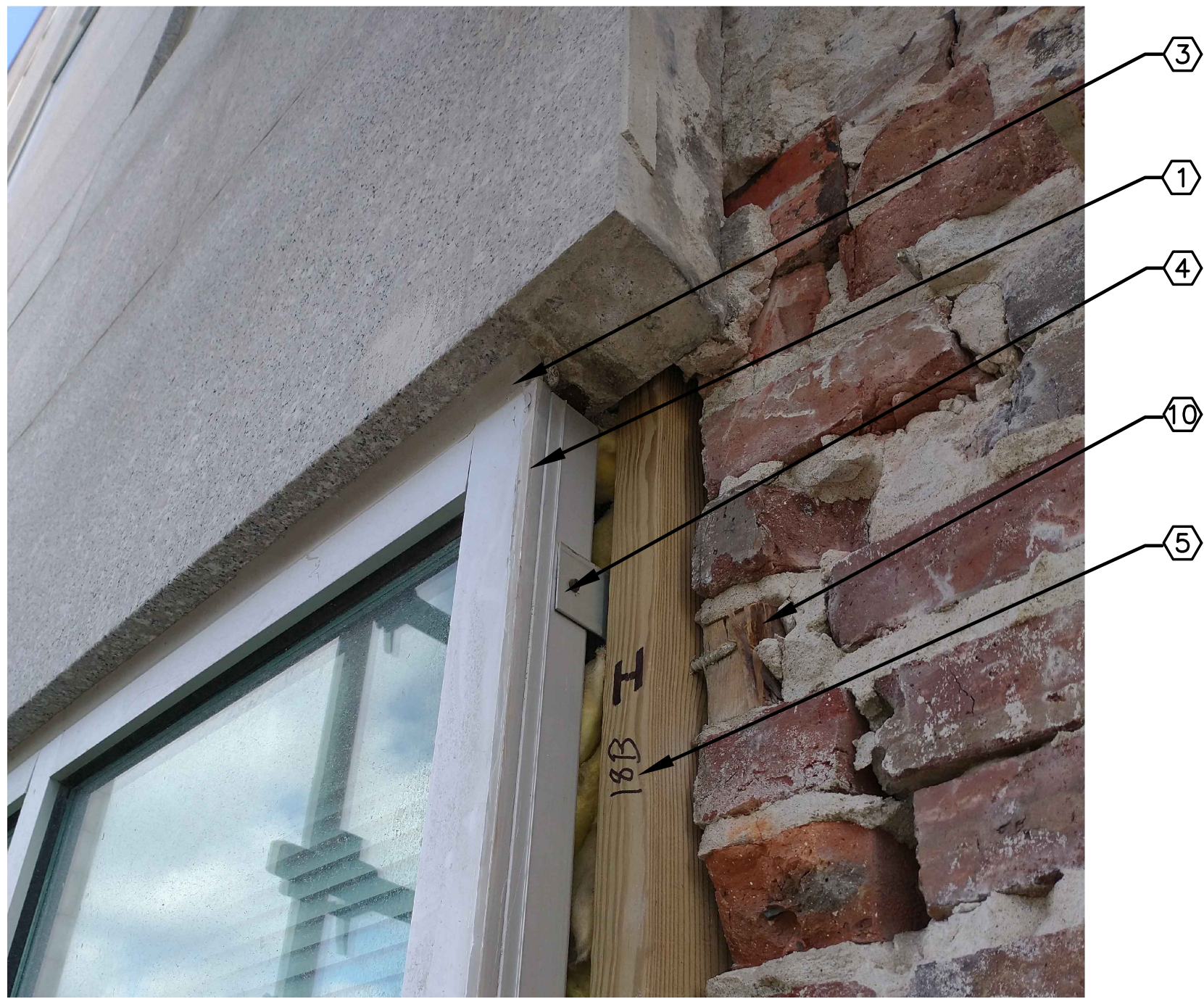
3 TYP WDW JAMB (GRANITE REMOVED) AD001/ NOT TO SCALE
