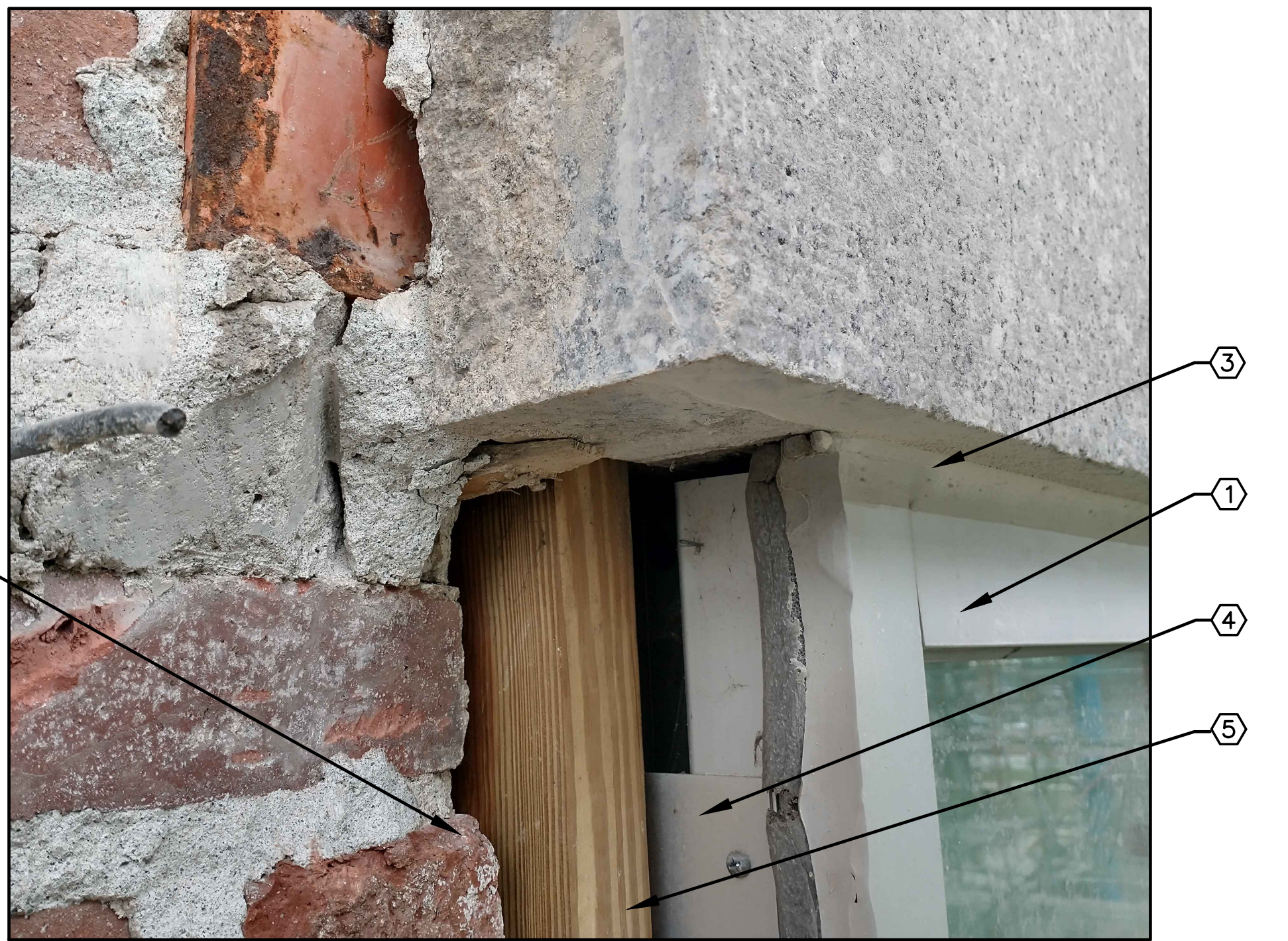
7 TYP WDW JAMB AT HEAD (GRANITE REMOVED) AD001/ NOT TO SCALE
