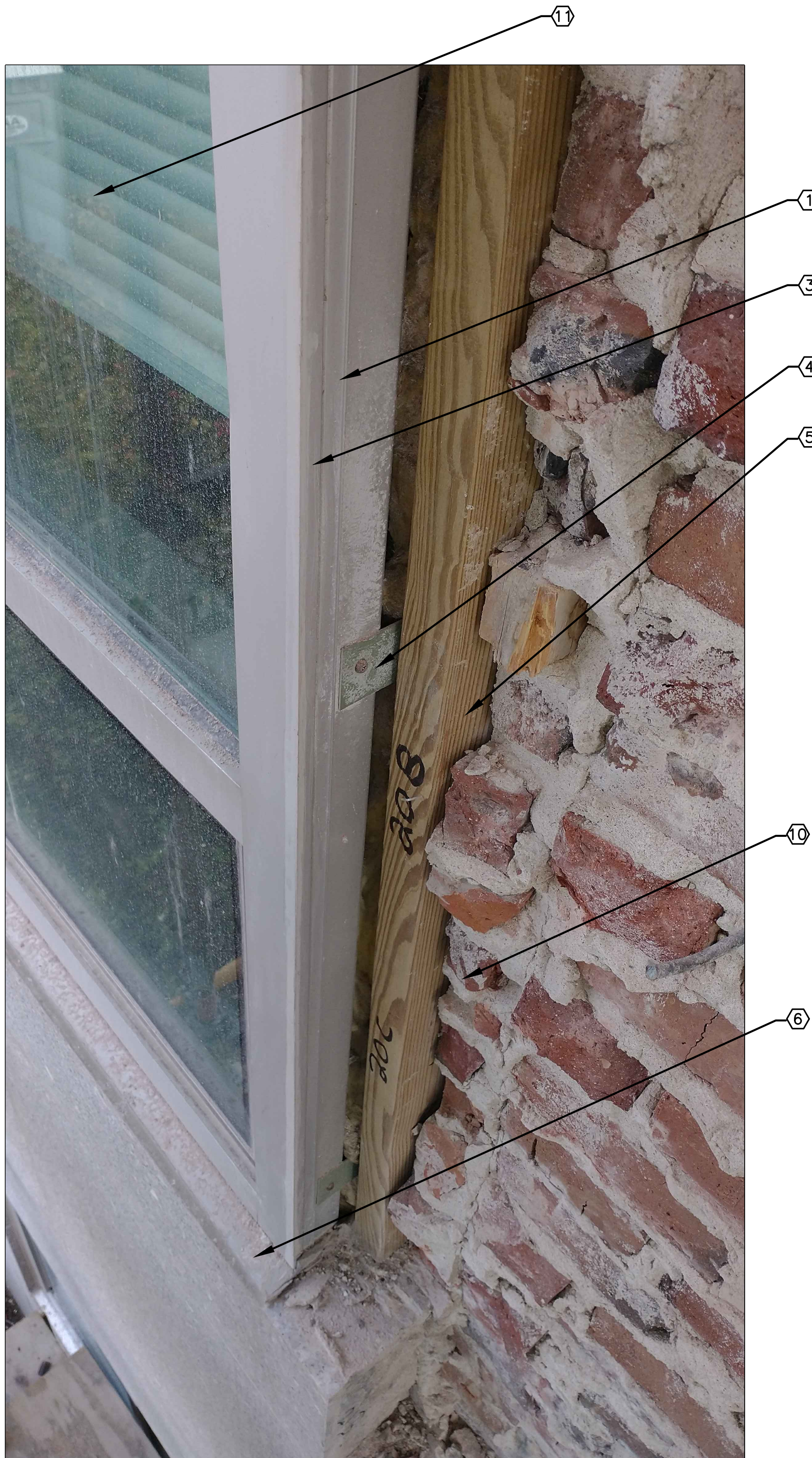
8 TYP WDW JAMB (GRANITE REMOVED) AD001/ NOT TO SCALE
