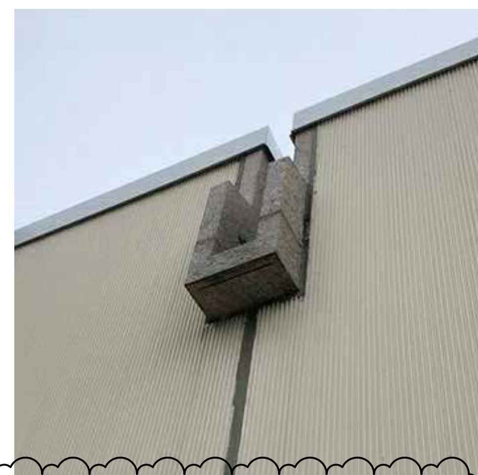
B4 PARGED CONC BASE 12" = 1'-0" NOTE THE DETERIORATING PARGING FINISH.
