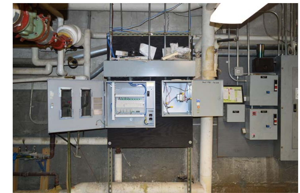
13 EXISTING SIEMENS RESET WATER CONTROLS TO BE REMOVED NO SCALE
