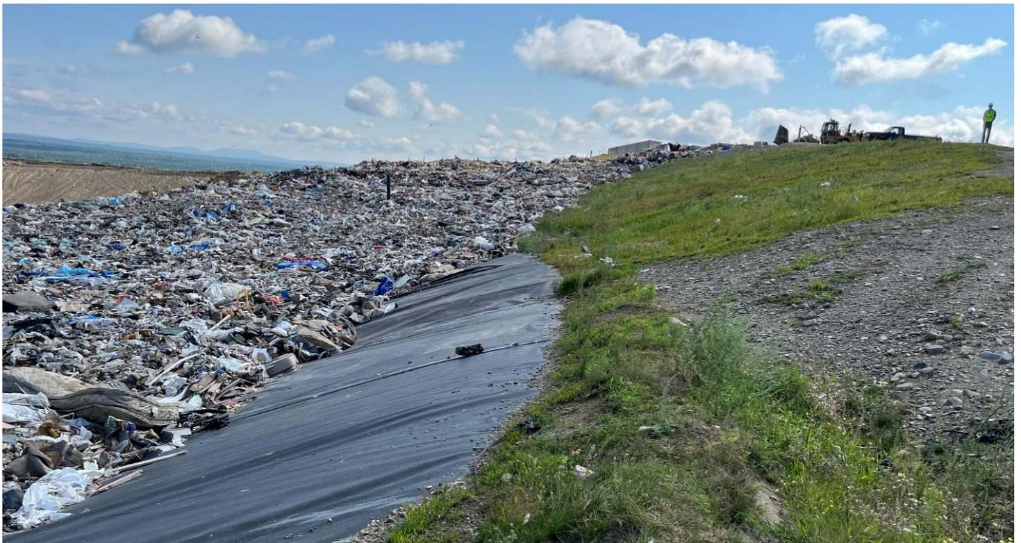
24. on top of Cells 3/7 looking easterly towards the placement of supplemental waste (to bring the settled northern slope of Cell 3 back to final grade)
