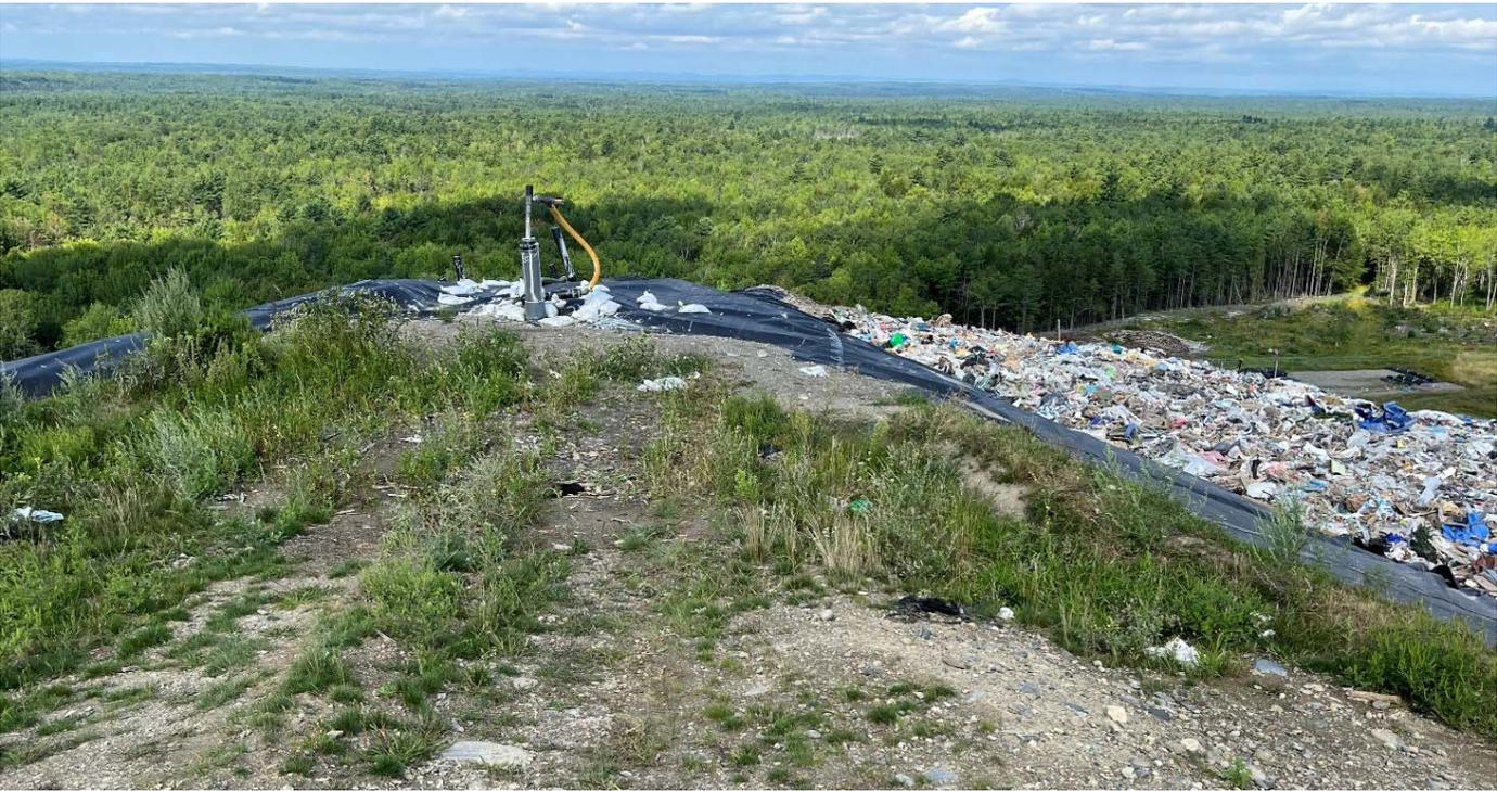
18. looking northwesterly down the top of the ridge formed on the northwest portion of the landfill (note right: supplemental waste placed to bring the settled northern slope of Cell 3 back to final grade)
