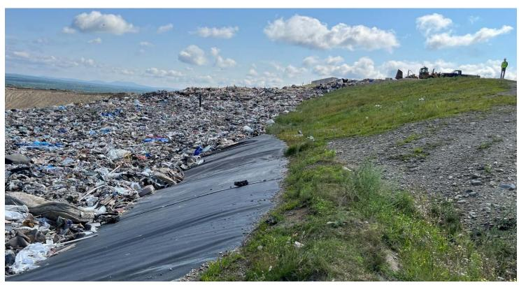
24. on top of Cells 3/7 looking easterly towards the placement of supplemental waste (to bring the settled northern slope of Cell 3 back to final grade
