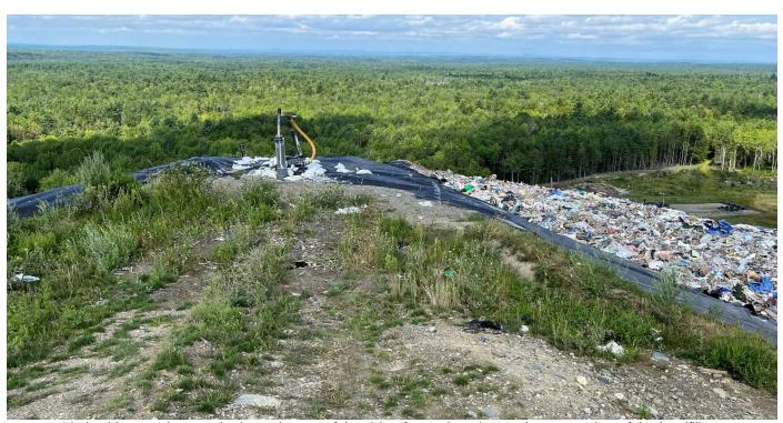
18. looking northwesterly down the top of the ridge formed on the northwest portion of the landfill (note right: supplemental waste placed to bring the settled northern slope of Cell 3 back to final grade)
