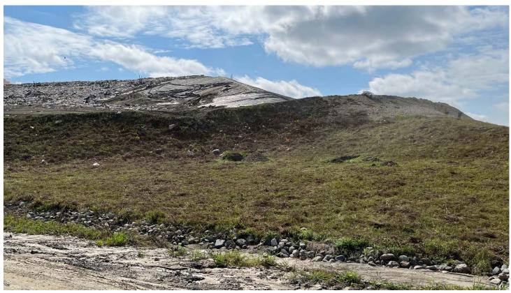
41. at northwestern toe looking up closed Cells 2/1 & waste placement at top of northern slope
