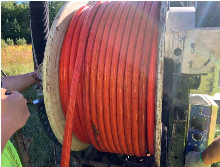
Clean Line at Manhole 13
