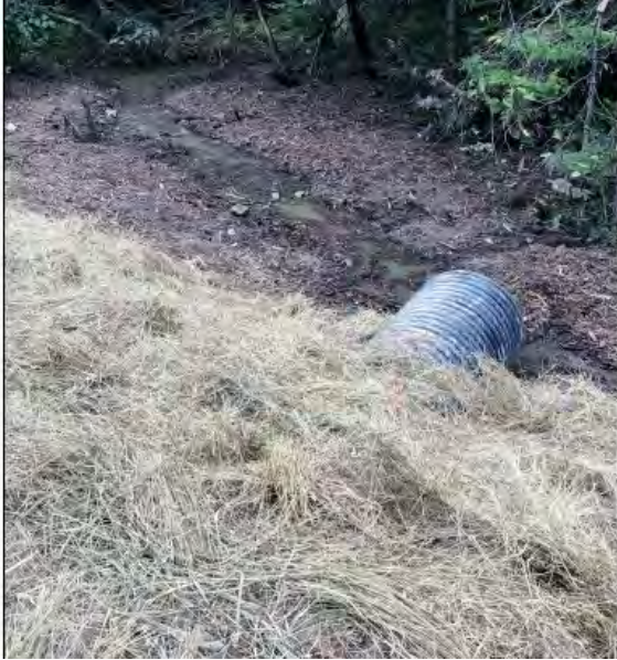
Upstream end of culvert after replacement (9/12/2020)
