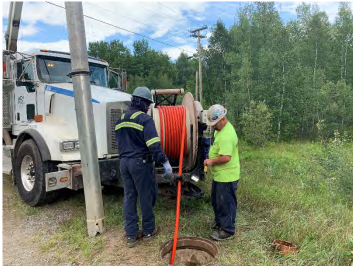
Cleaning at manhole 4
