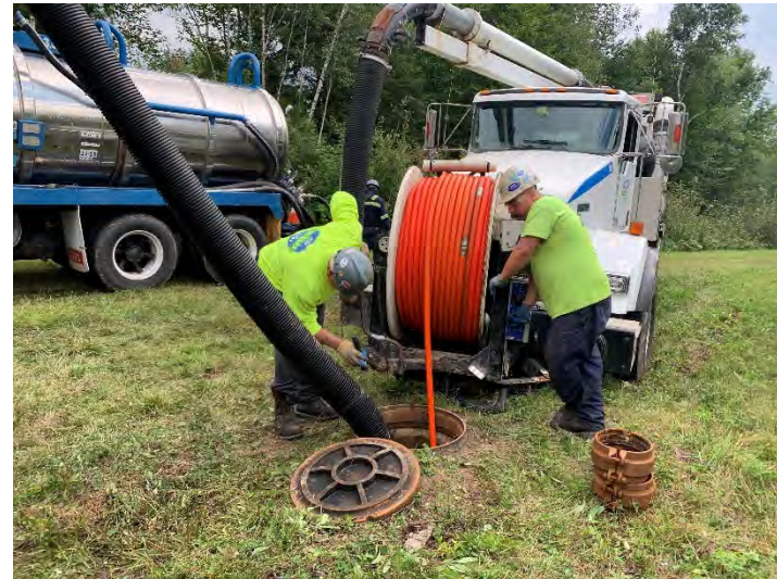
Cleaning at manhole 5
