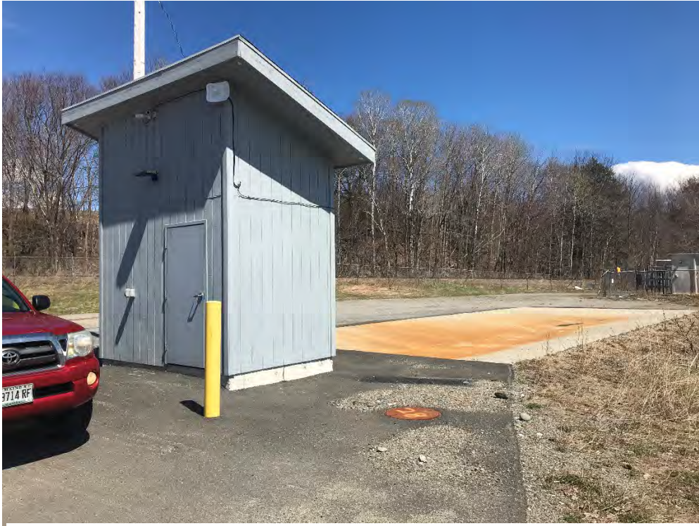
Leachate Pipeline Flow Meter Building and Emergency Leachate Unloading Pad
