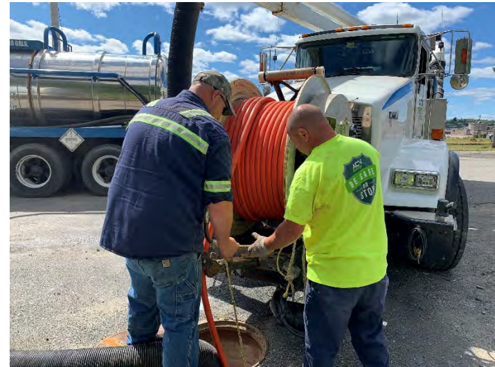
Cleaning at Manhole 17
