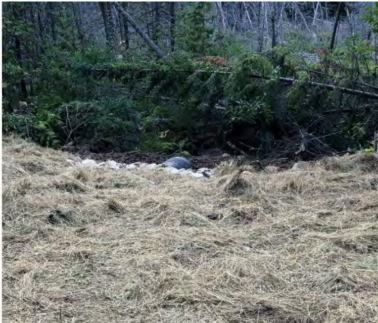
Downstream end of culvert after replacement (9/12/2020)
