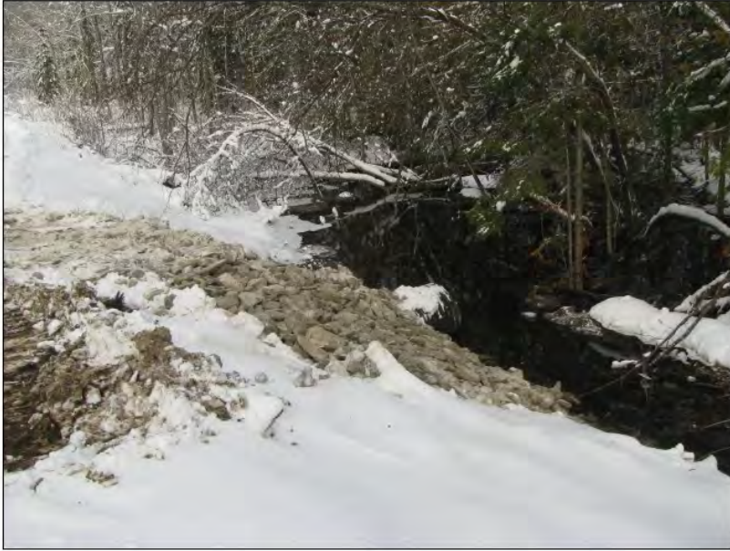
Upstream end after riprap placement (12/9/2020)
