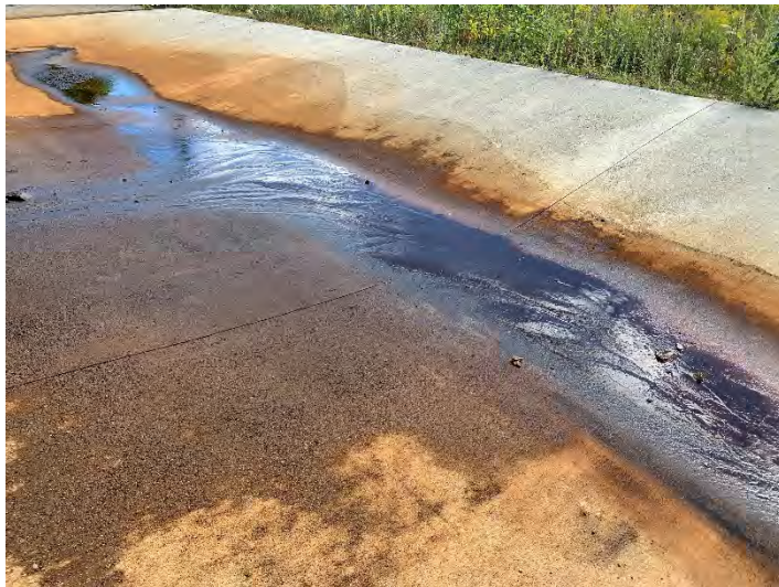
Sediment on leachate dumping pad after cleaning from manhole 23 to manhole 26
