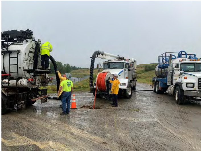
Cleaning at manhole 2
