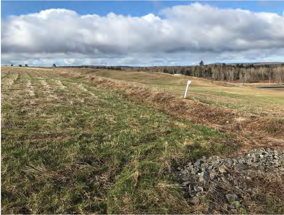
Dolby III Cover Upgrade Area (West Side)
