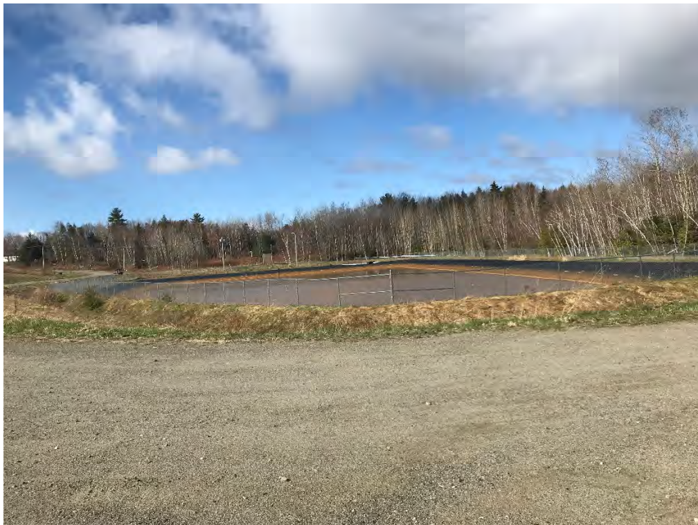
Dolby Leachate Pond
