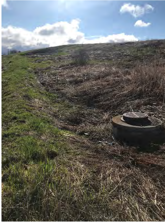
Dolby III Open Area (North Side)
