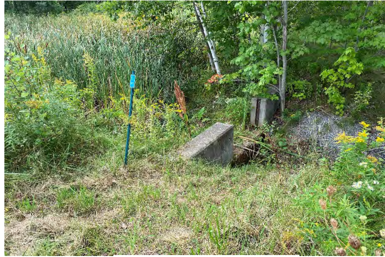
West Sediment Pond Outlet
