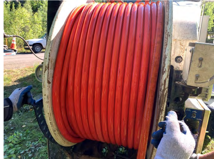
Clean Line at Manhole 11
