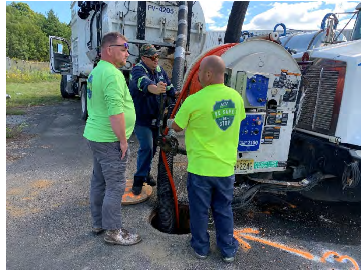
Cleaning at manhole 23
