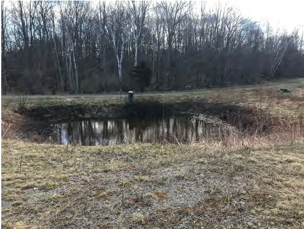
Dolby II Leachate Holding Pond
