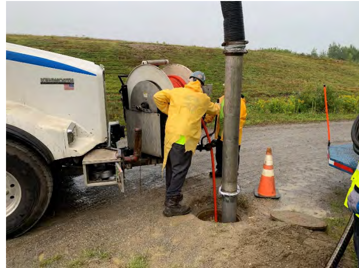
Cleaning at manhole 2
