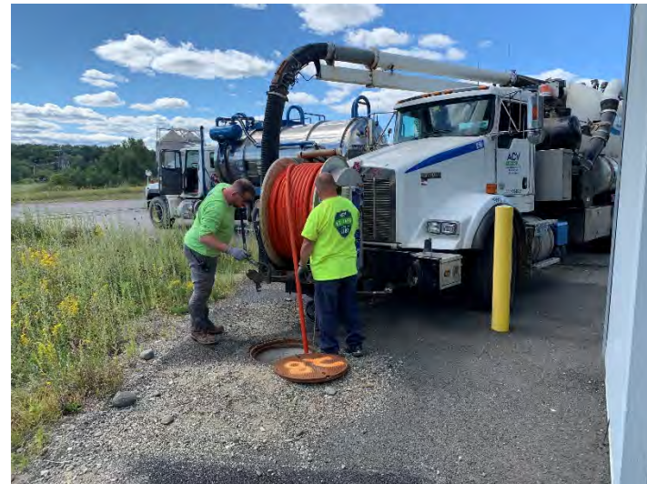
Cleaning at manhole 28
