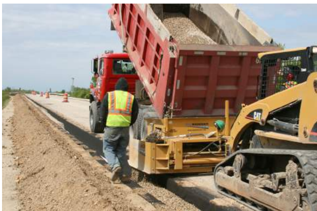
Trenching using the Road Widener.
