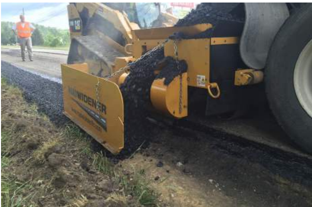
Laying down asphalt using the Road Widener.
