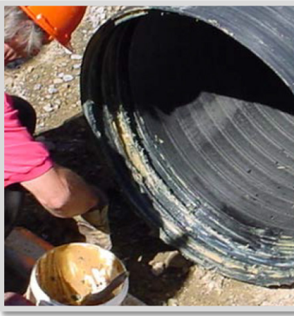
Step 1: Prior to threading pipe, grease the threads to reduce the threading force required.
