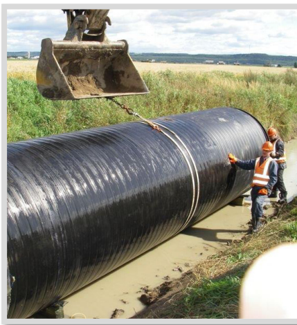
Step 3: Use nylon slings with lever or excavator arm to rotate the pipe.
