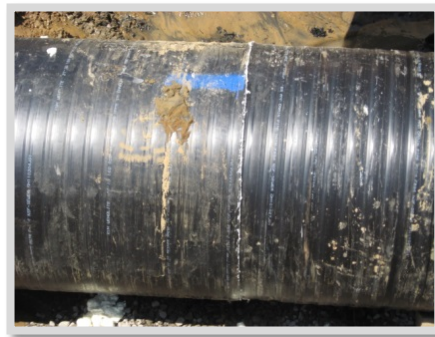
Step 4: Wipe off excess foam if necessary.
