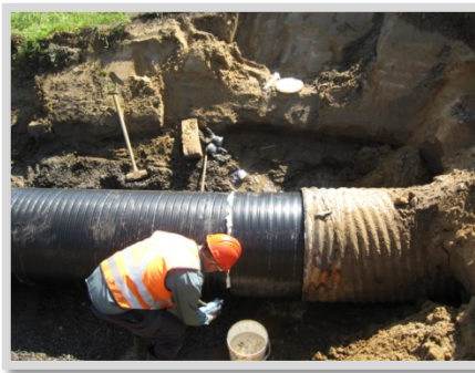
Step 3: Finish spinning the threaded joint until thread will not spin anymore.
