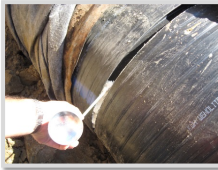
Step 1: Thread pipe together until 1 complete turn is remaining to complete threading.
