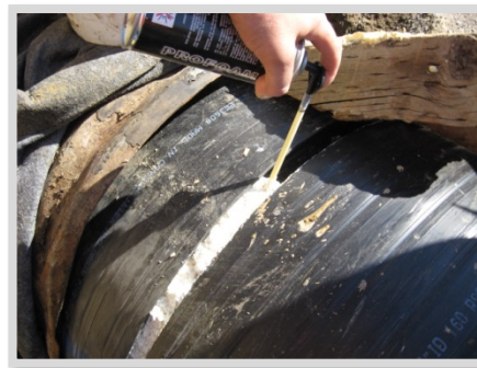
Step 2: Using closed cell polyurethane spray foam, spray foam in joint around entire circumference of the pipe.
