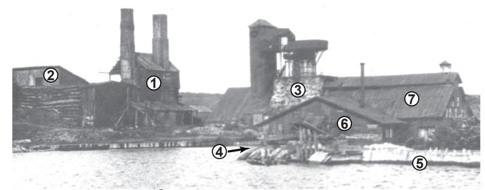
While ore was roasted in the Iron Kiln①workers filled the Charcoal Storage Shed②with charcoal from the brick kilns. The charcoal, ore, and limestone were dumped into the Furnace③and then superheated by pumped-in air. A Sluiceway④ diverted water from the Dam⑤through the Machine House⑥where it powered cylinders that forced the air into the furnace. The melted iron then ran out into sand molds on the floor of the Casting House⑦where the pigs were formed.
