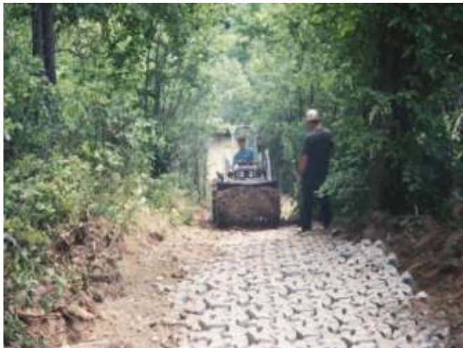
After the blocks are in place cover them completely with fill to a depth of about 2 inches.
