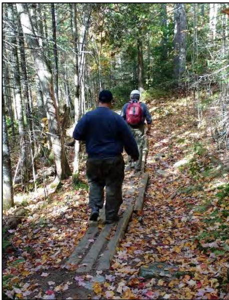
Bog bridging on the Holeb portage trail.
