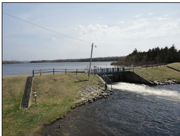
West Outlet dam.
