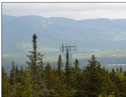
Communications Tower on Bald Mountain Unit
