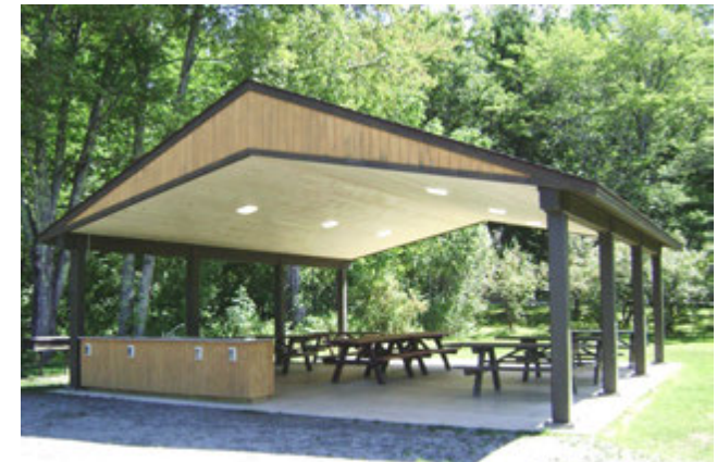
Group Shelter, Damariscotta Lake State Park
