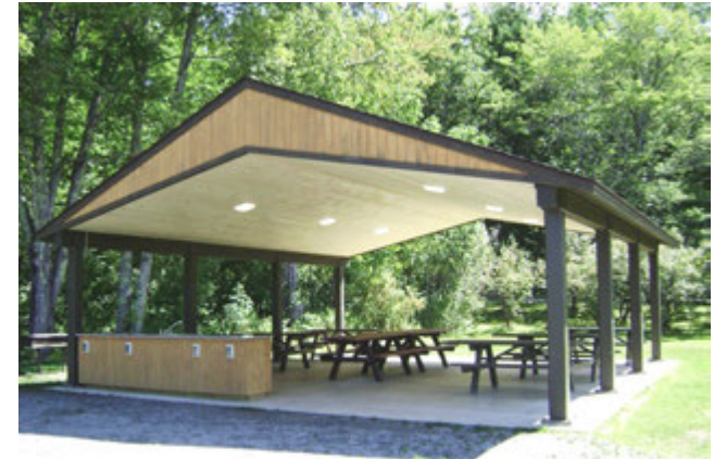
Group Shelter, Damariscotta Lake State Park
