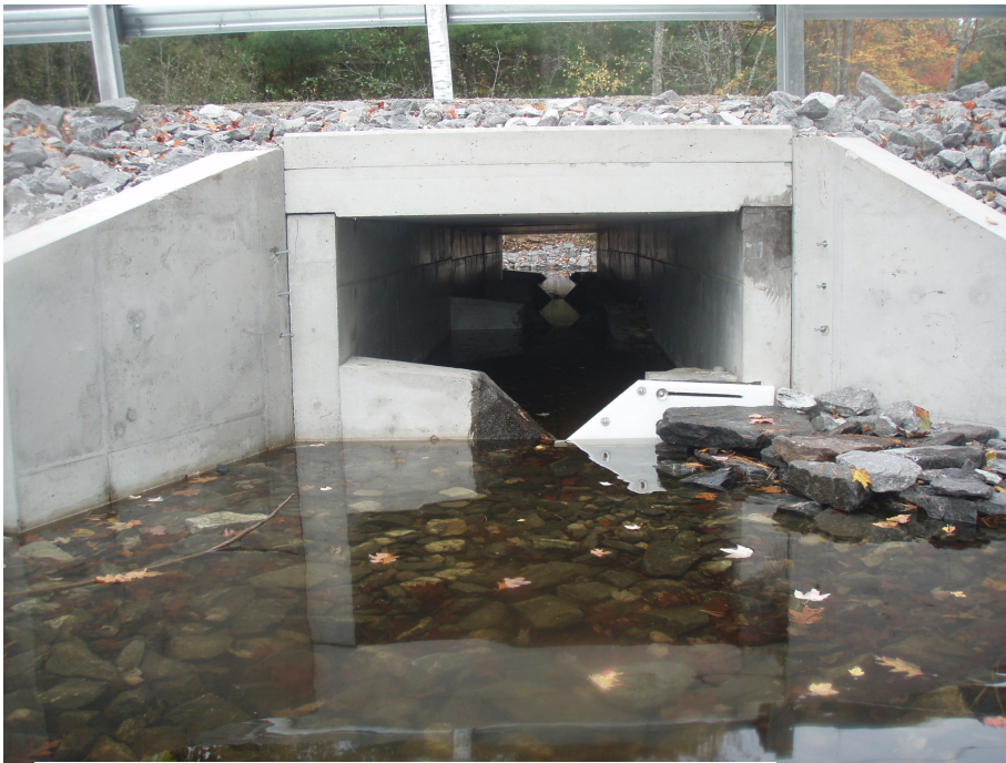
Figure 6.7 Box Culvert at Sewell Pond in Arrowsic
