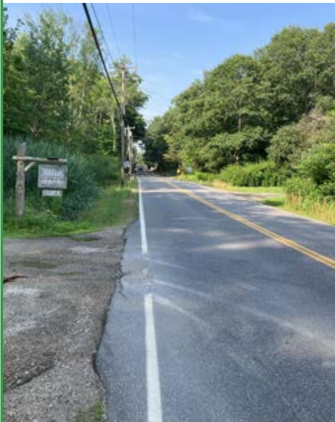
Beech Rd. looking toward State Rd. (July 2023). The road, which connects the Village area with Eliot Commons and Route 236, lacks a sidewalk and shoulders, meaning people must walk on the dirt shoulder, in the ditch, or in the travel lane.
