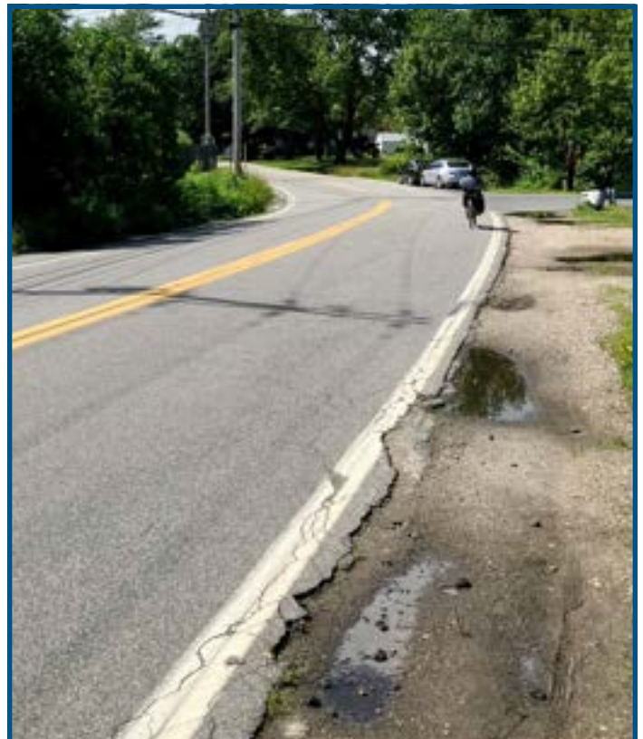
A person riding a bicycle in the travel lane of Main St. near Bolt Hill Rd. Deteriorated roadway edges can present a hazard for people on bike.
