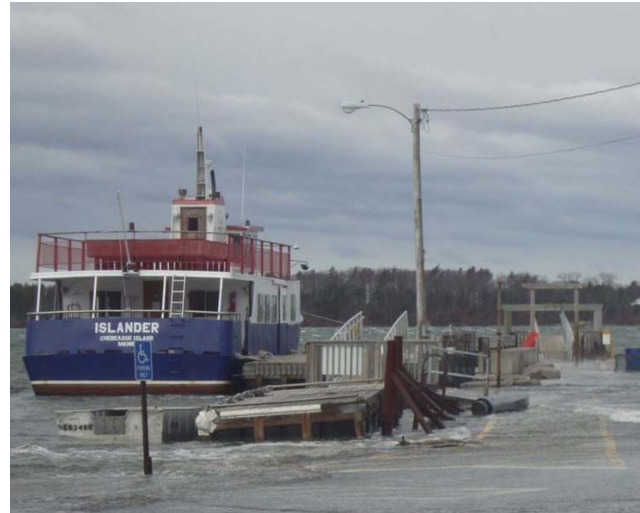
Inundation of Chebeague Island's Stone Pier
