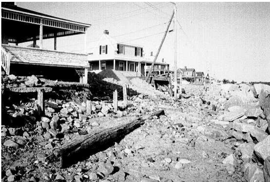
Figure 2. Erosion and property damage at Camp Ellis.
