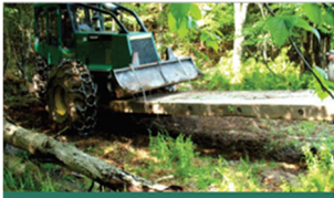
INSTALL BRIDGE PANELS
