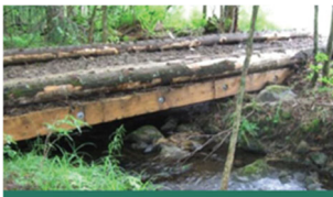
INSTALL BUMPER LOGS
