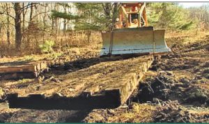
REMOVING THE BRIDGE
