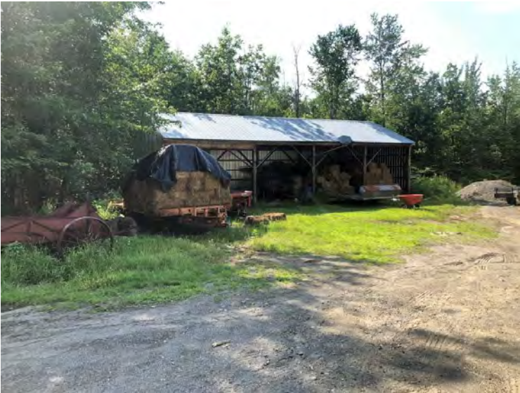
Photo 7 – Andrews property. View west toward the pole barn constructed on recently-filled wetland.
