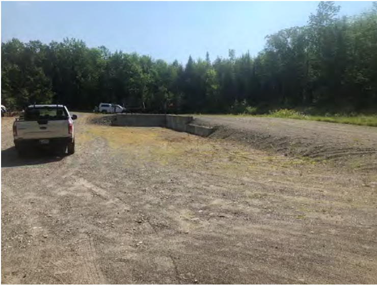
Photo 1 – Russel property. View east of the building pad constructed by the landowner.
