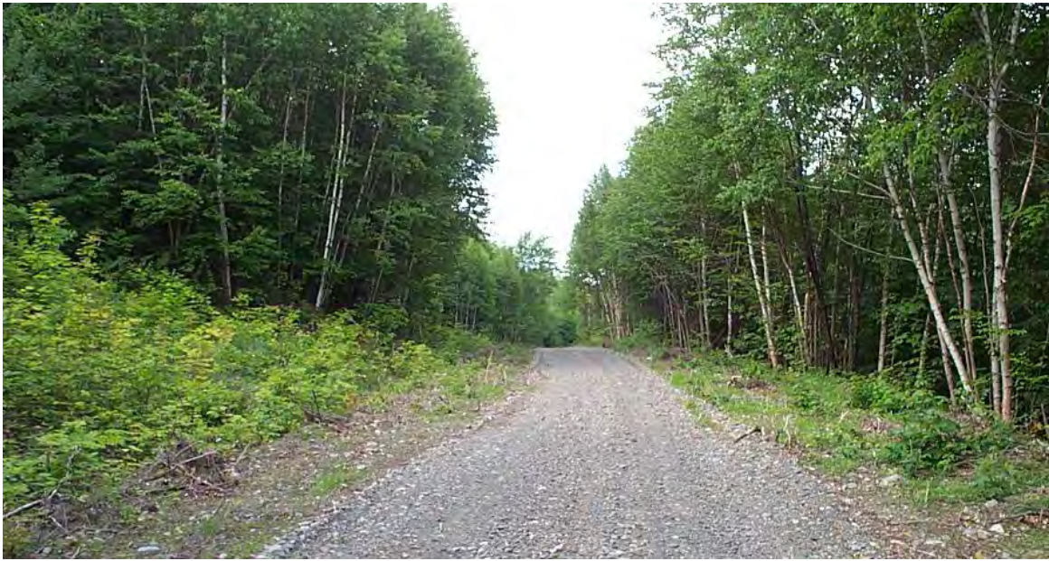
Foss Pond - Access Road West Side
