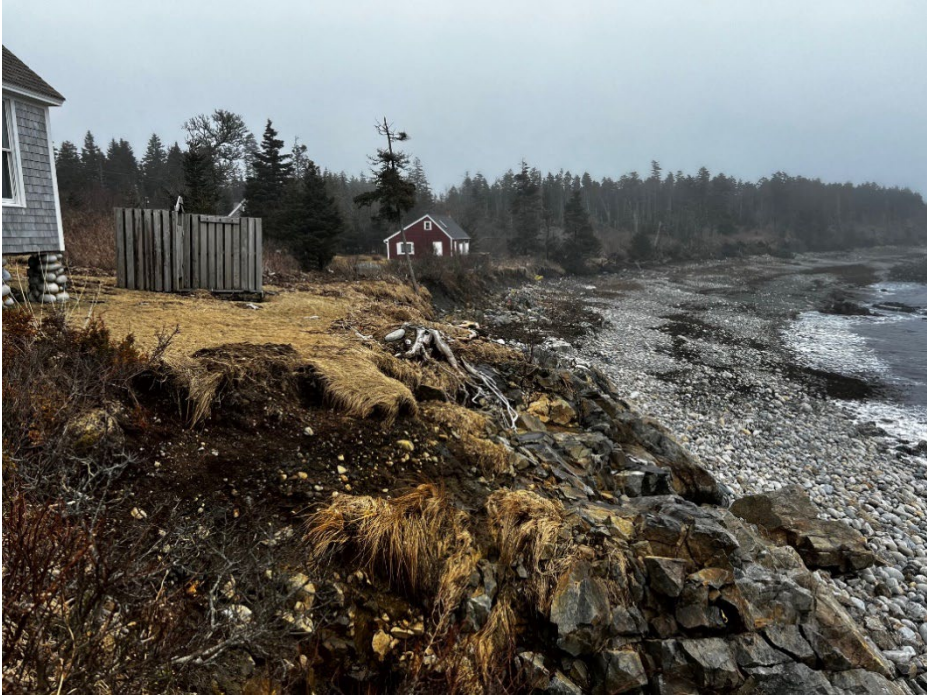
Shoreland Erosion, Matinicus Island
