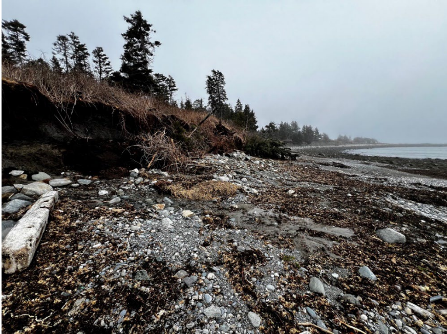
Shoreland Erosion, Matinicus Island
