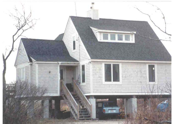
Elevated home in Georgetown, Maine. Photo by Bonnie Cowle, Maine Floodplain Management Program
