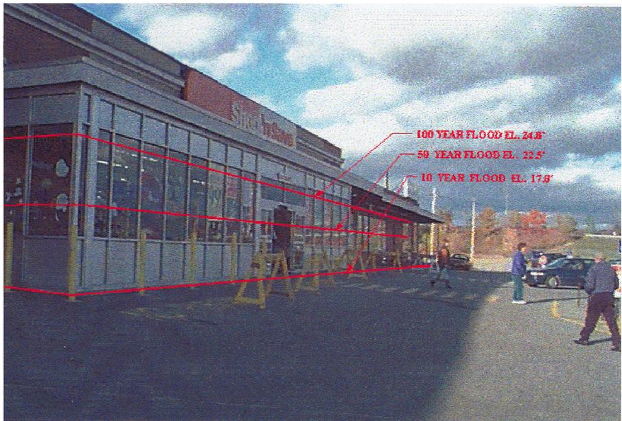
Flood Levels at Gardiner Shop 'n Save, from the 1994 FEMA flood insurance study. 10 year flood level is at the existing ground floor of Shop 'n Save, 50 and 100 year flood levels cause 5.5 feet and 8.8 feet, respectively, of water above the floor. The 1987 flood was a 100 year flood.
