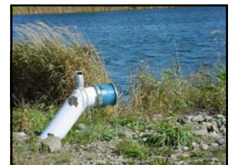
Permanent irrigation intake structure.
