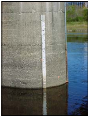
Aroostook River water level gauge.
