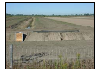
Cranberry bog construction.
