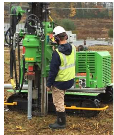
Ground Screw Installation Source: ReVision Energy
