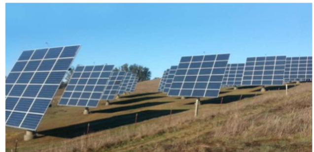
Tracker solar farm utilizing concrete piers
