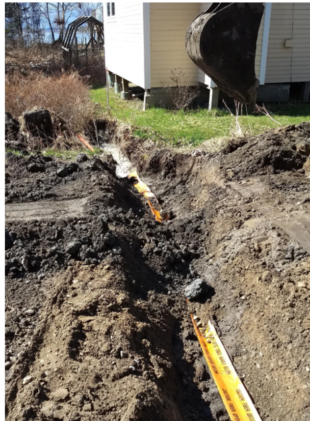
Fiber being laid on Cliff Island (Courtesy: Nate Brimmer)
