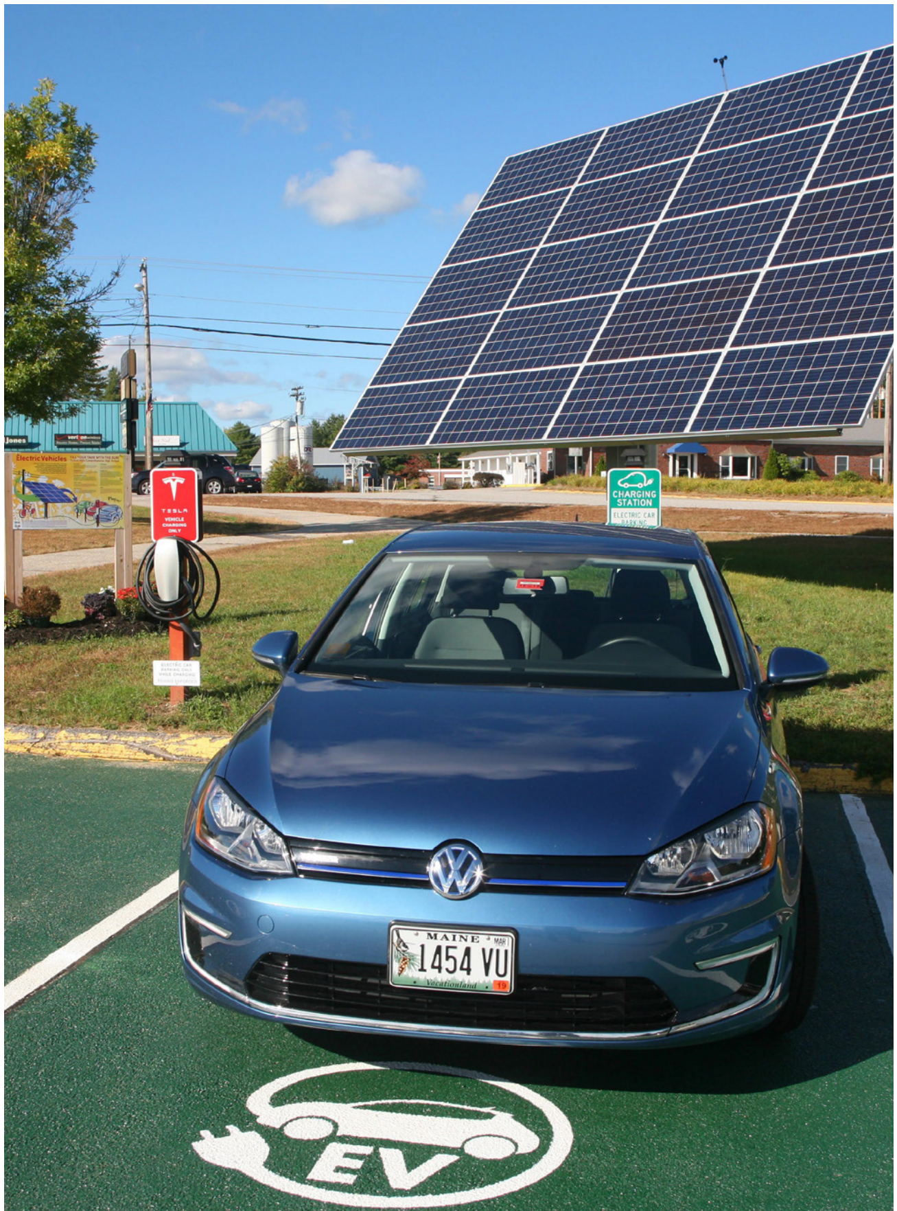
Solar panels power these EV charging stations at Oxford Hills High School in Norway.
