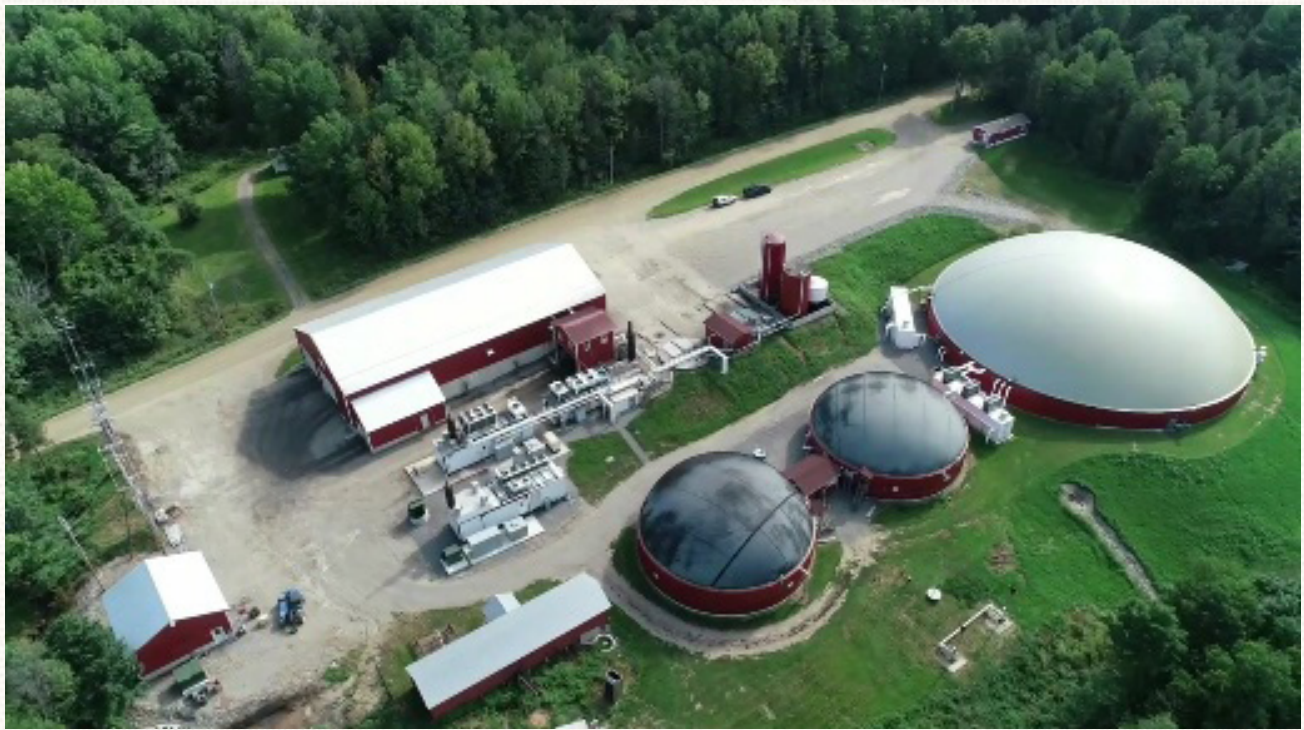
The digester facility at Agri-Energy in Exeter processes food waste to extract methane gas for energy on a continuous 24/7 system.
