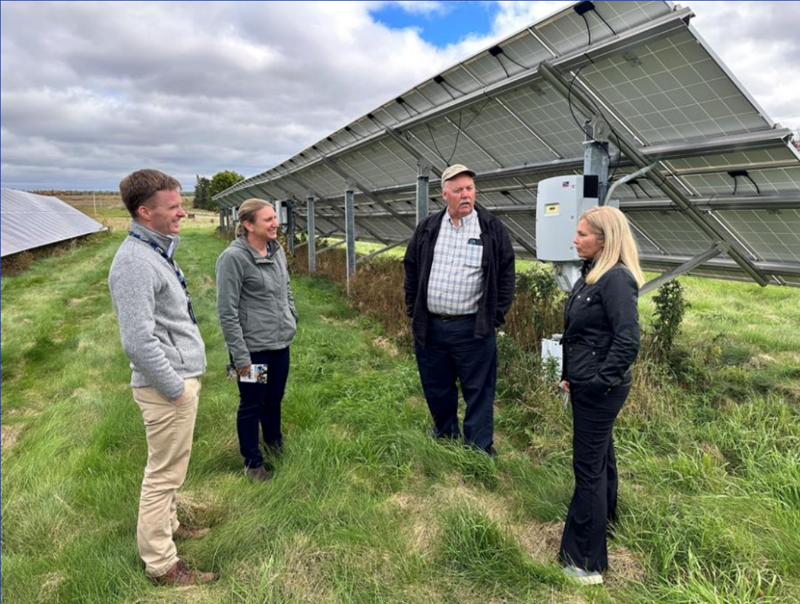
Community Solar project in Limestone, Maine
