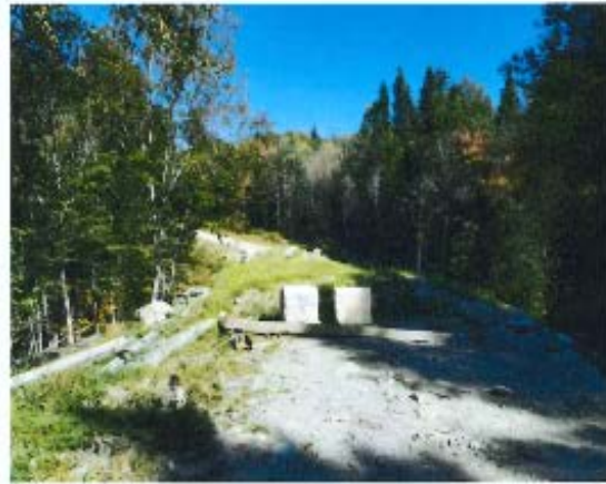
Approach Heading North
