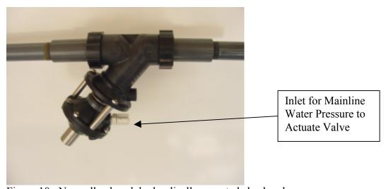
Figure 10: Normally closed, hydraulically operated check valve
