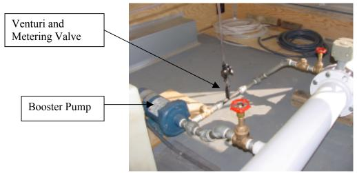
Figure 7: Venturi installed in bypass configuration
