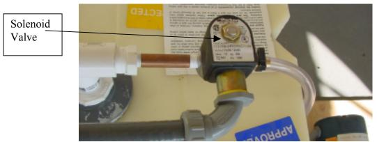
Figure 3: Normally closed solenoid valve
