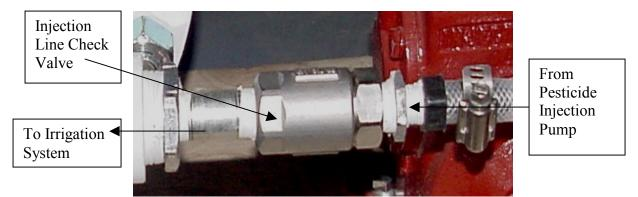
Figure 2: Quick-closing check valve on pesticide injection line
